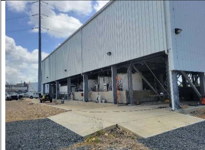
Picture 19 View of the WWTP.
