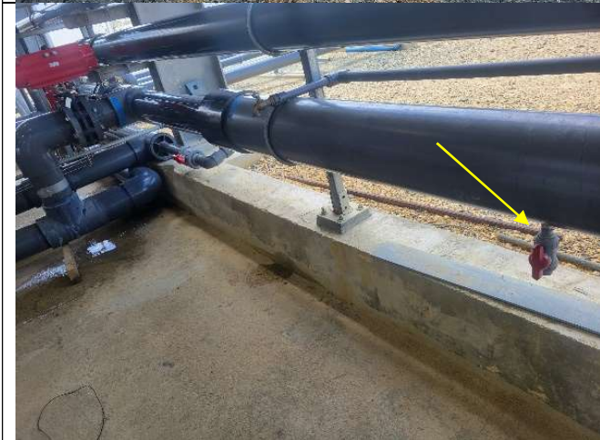
Picture 20 The yellow arrow depicts the location where samples will be taken. The flow meter is located after the red box.
