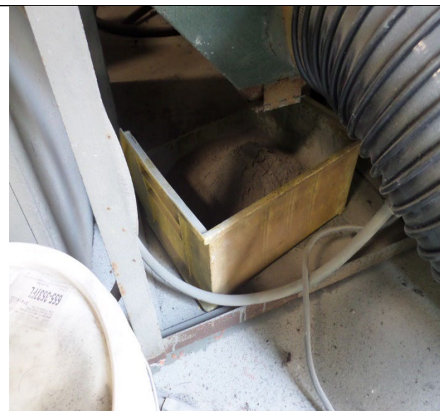
Chlorine Packaging. Blast Cabinet Area. Inspectors observed spent blast media in a small plastic tray and on the floor under the blast cabinet. Observed the blast cabinet was not operating and the container was open. Photograph 12 taken at 11:52 a.m.
