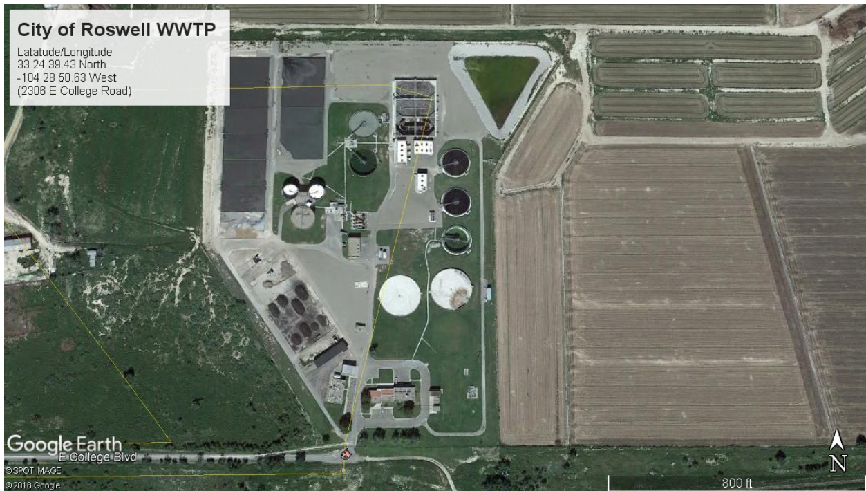
Aerial Image #1: Overall view of the City of Roswell’s Wastewater Treatment Plant. Aerial from Google Earth maps.
