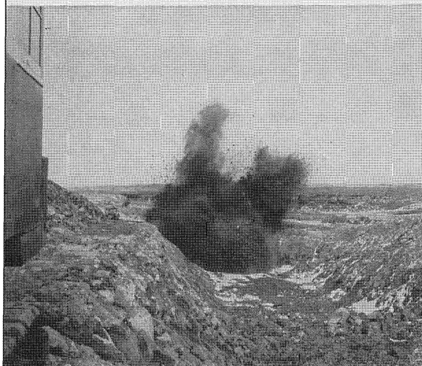
Common use of Du Pont dynamite on project is in ditching and tunneling to drain surface water that collects each autumn.
