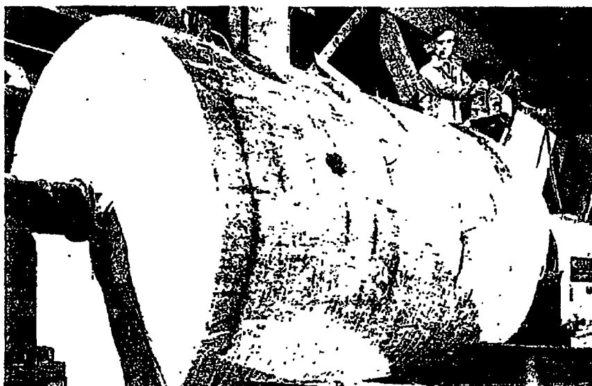
Giant Douglas Fir log in lathe ready to be peeled into plywood veneer.
