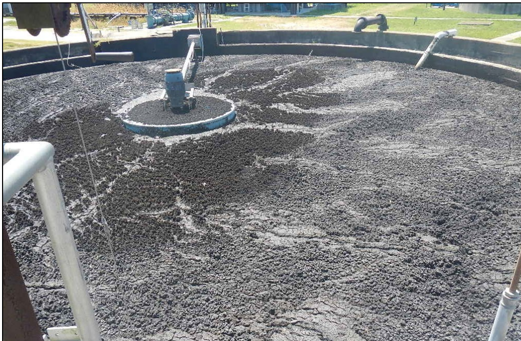
Photo 8. Final digester basin.
