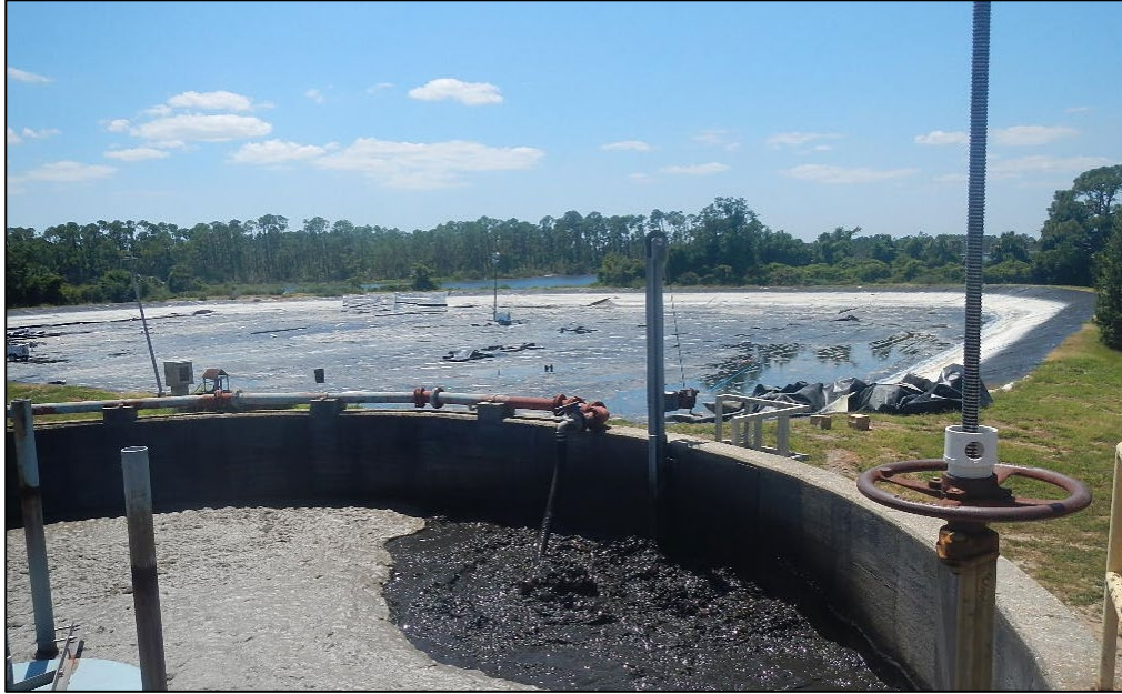
Photo 7. Digester basin and the reject pond in the background.
