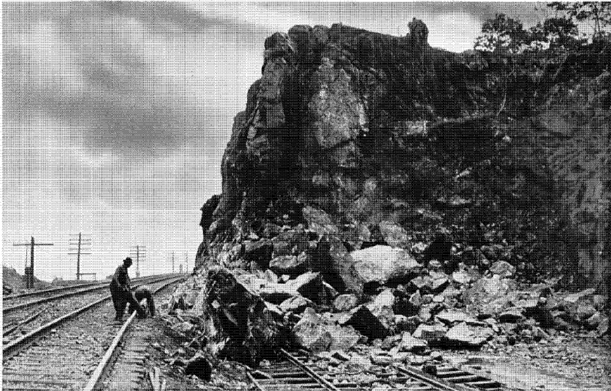
A view of the south end of Beverly cut, north of Manitou, New York. The ledge of rock, averaging from 60 to 80 feet in height, is being cut away for a distance of almost a mile. Note the proximity of operations to the main-line tracks.
