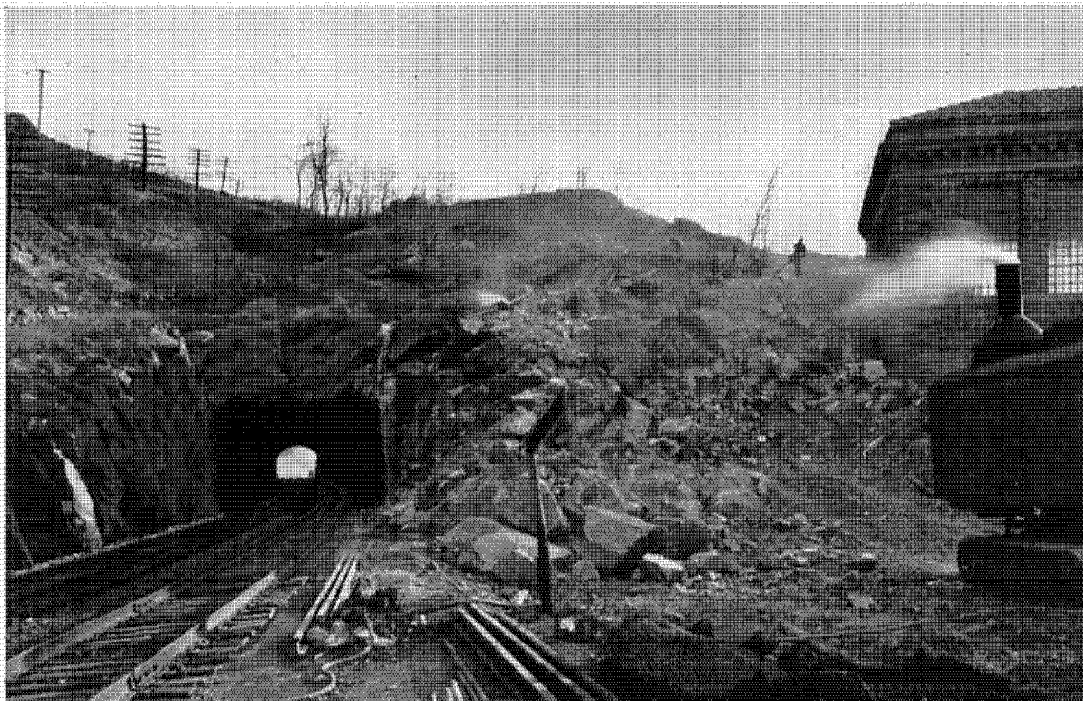
This view of the old Breakneck tunnel was taken before the work of driving the north portal of the new tunnel had started. Its location may be seen in illustration 2 on the preceding pictorial page
