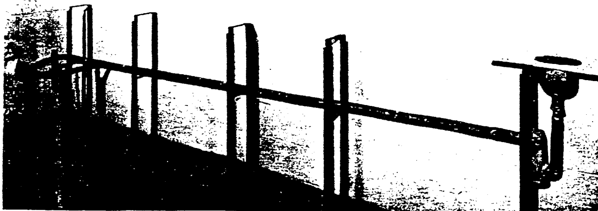
Another of the many lead waste lines from the lead cup sinks in chemical laboratory tables installed in the new wing of the University of Arkansas' Medical School.
