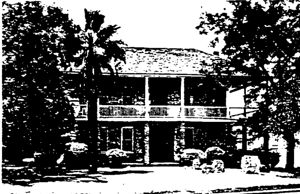
"Houston's oldest landmark. Noble House, is steeped in early history. Worth seeing."
