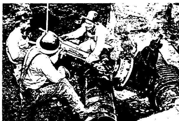
JUNE—The plant pipelitters made a difficult job look easy early last summer. There was a need for another cooling water outlet off the water main picture here, and J. F. Flynn, J. F. Grubbs and C. E. Sharp promptly "shot-tapped" the main with pressure remaining in the water system throughout the operation.
