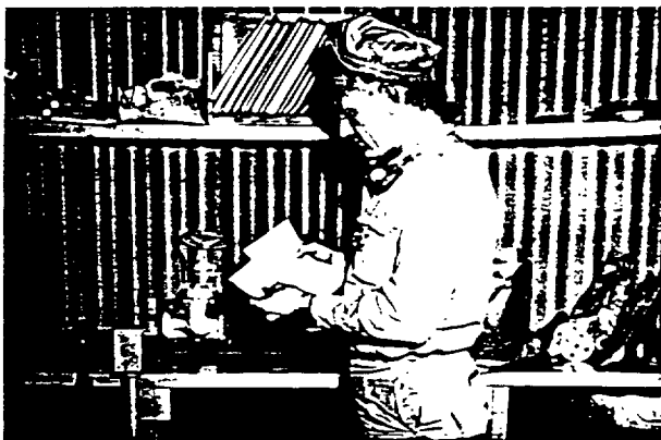
ROUND ROBIN —Here the valve ordered by Ferguson is delivered to the Receiving Station by Fannin. The original Store Order is picked up and attached to the withdrawal slip written up by the "phoneman." These forms are returned to Stores Office for processing.
