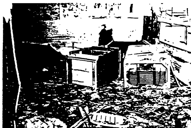
Some of the debris and foreign matter which swept into the Otis home is visible here in foreground. Lying on its side is a refrigerator, total loss.
