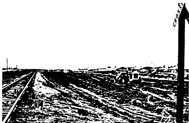
WORK UNDERWAY —This illustration shows roadwork near Deer Park being performed, and when the work is complete the railroad tracks will be moved to make room for the new LaPorte-Pasadena Freeway. At far left may be seen the present LaPorte highway.
