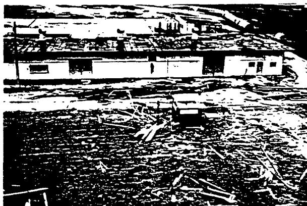
This area, far from the Ship Channel, shows evidence of debris and roofing deposited helter-skelter. A big cleanup job in all areas of the plant followed closely on the heels of the storm.
