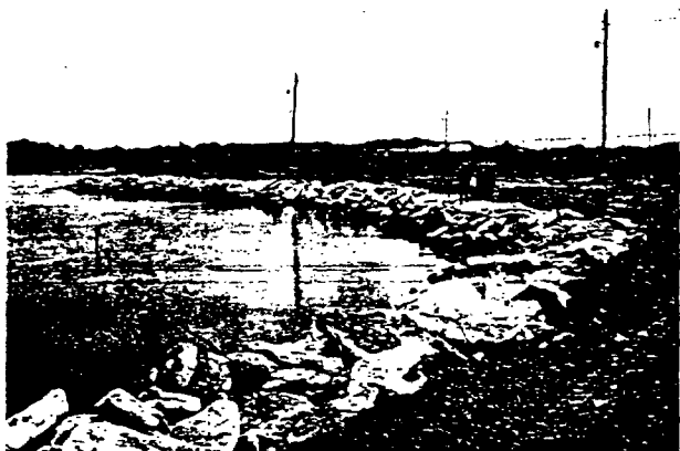
COMPLETED JOB —Shown here is about 700 feet of rip rap in place at the Ship Channel, complete except for smoothing the dirt approaching the rip rap, later to be planted in grass seed. Viewing the job from left are Bob Marshall, Benny Duke and Jack Knoone.
