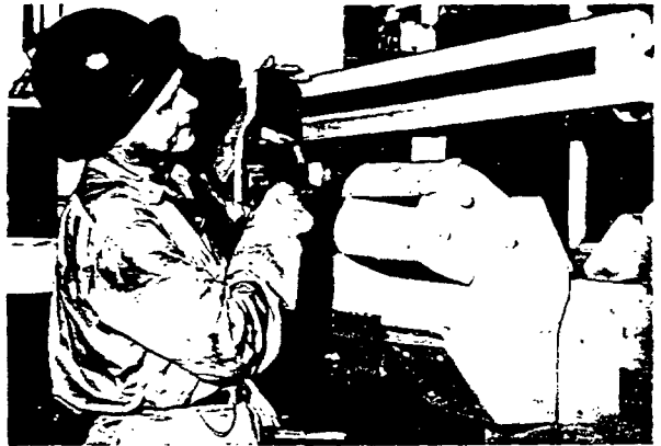
SCALE HOUSE WORK— Here Renfro disassembles the scale poise for an examination of the movements within this unit. The entire mechanism within the 50-foot scale pit below transmits minute movements of this beam, thus providing the reading upon which our customers are billed for products shipped. Perfect working condition of the scales at all times is a must.
