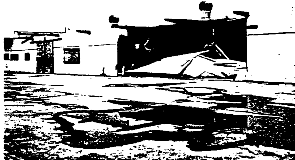
The south side of the old construction warehouse, near Garage, shows some effect of the strong winds which occurred Monday, September 11. Only superficial damage was sustained on permanent installations.
