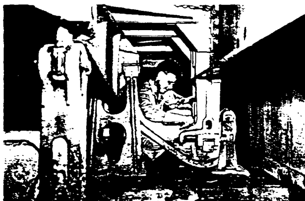
DEEP IN THE HEART OF— Tom Renfro, outside machinist, who is responsible for plant scale maintenance, is shown here in a track scale pit. He is probing into one of the pivots on this scale for harmful dust deposits which can adversely affect the movements when a load is being weighed. The track scale pits are steam heated to drive off moisture.
