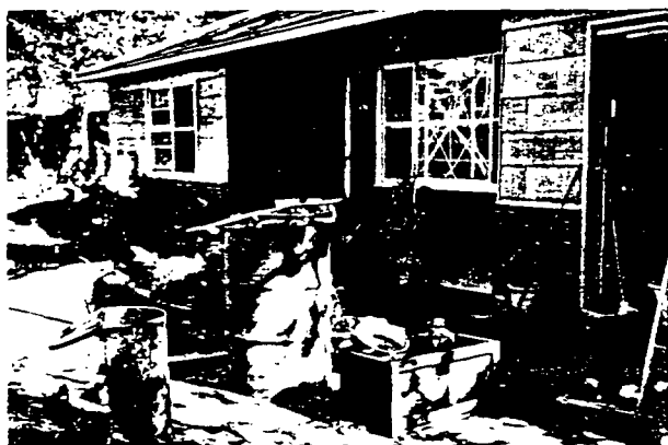
Operation cleanup. Every available container is filled with the debris hauled out of the house—once treasured family possessions.
