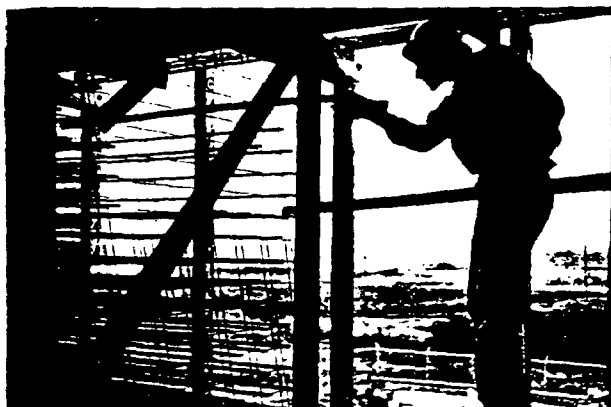
OCTOBER —A real "cool" job undertaken last fall was the replacement of baffles in the water tower. This unique view shows Carpenter Joe Baltuskonis easing new baffles into position. There are about 9,000 slats in each of the four sections of the cooling tower.
