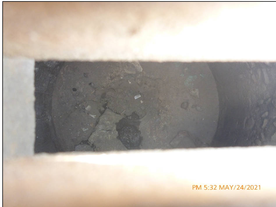
Photograph 11. View of inside the catch basin of the Outfall 005 storm drain.
