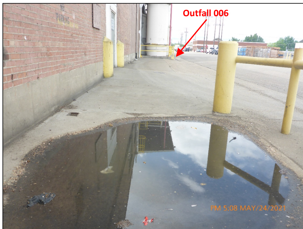
Photograph 14. View of the accumulated stormwater shown in Photograph 13. This portion of the Facility discharges to Outfall 006 shown in Photograph 12.
