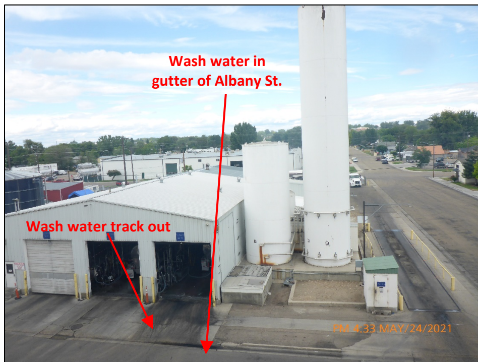
Photograph 26. View, facing northeast from the main production building rooftop, of the milk tanker loading/unloading building on the northeast side of Albany St. (eastern parcel). Note the wash water track out and accumulated wash water in the gutter line of Albany St.
