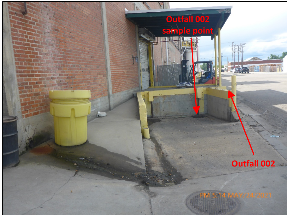
Photograph 7. View, facing northwest, of the loading bay storm drain that flows to Outfall 002. Samples for Outfall 002 are collected from the catch basin of this loading bay storm drain.
