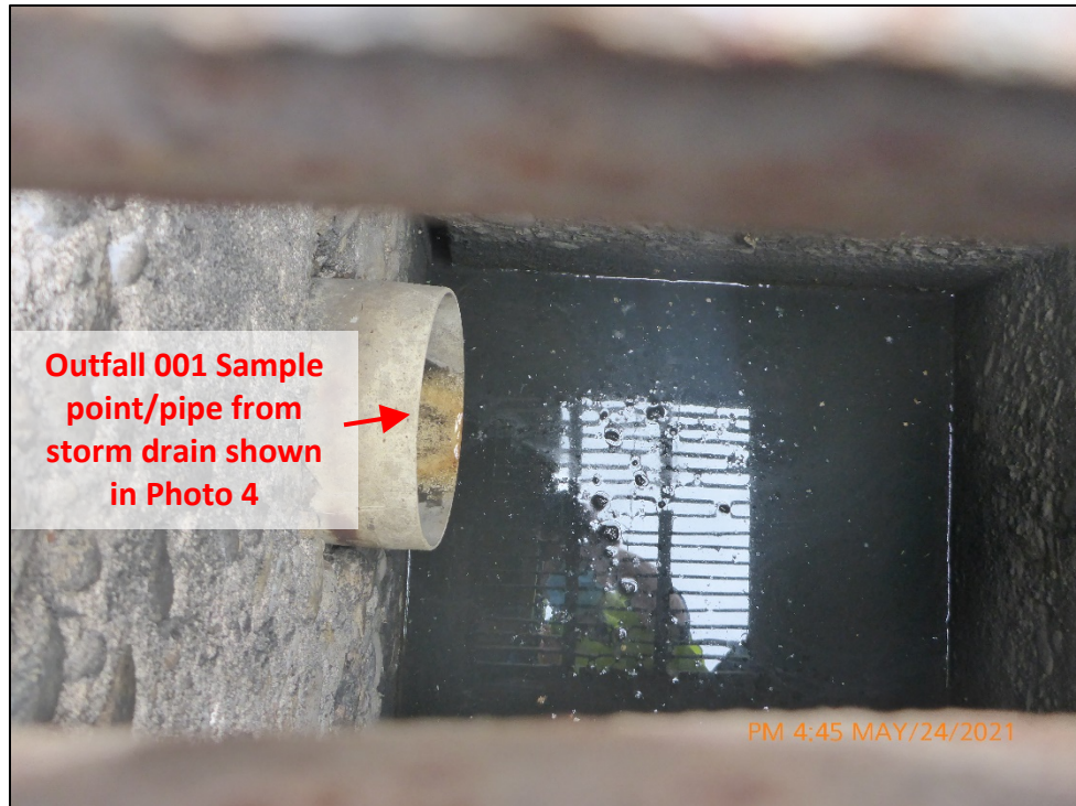
Photograph 3. View of the PVC pipe into the Outfall 001 storm drain catch basin where compliance samples for Outfall 001 are collected.
