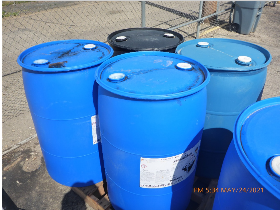
Photograph 36. View of empty 55-gallon drums stored outside near the wastewater treatment system and Outfall 005. Note one of the drums did not have a bung cap in place.
