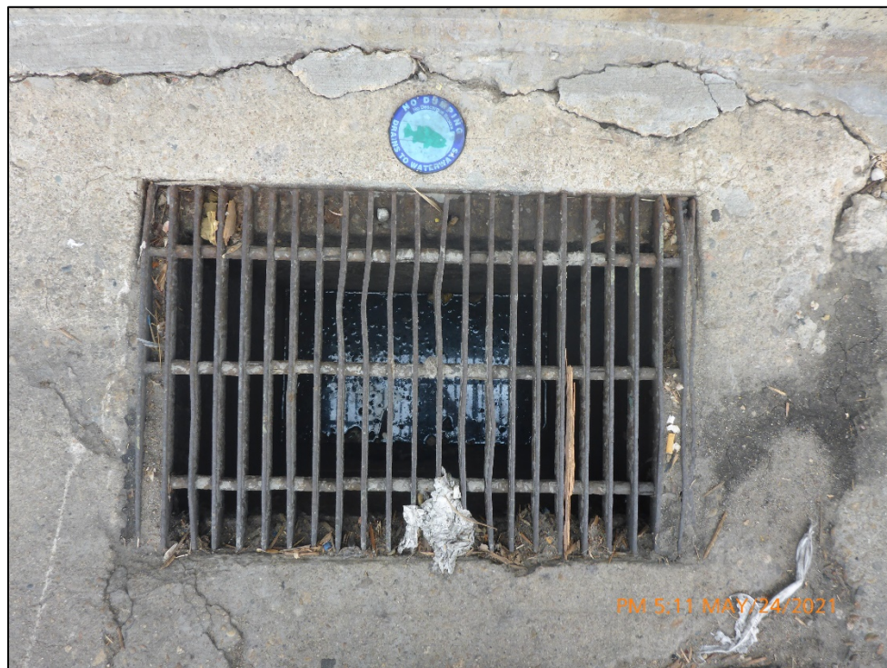
Photograph 6. Close-up view of Outfall 002.
