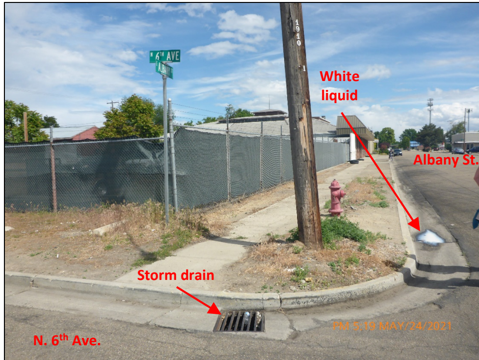
Photograph 19. View, facing east, of a storm drain inlet at the east corner of Albany St. and N. 6 th Ave. Note the white liquid in gutter line of Albany St. upgradient of storm drain inlet.
