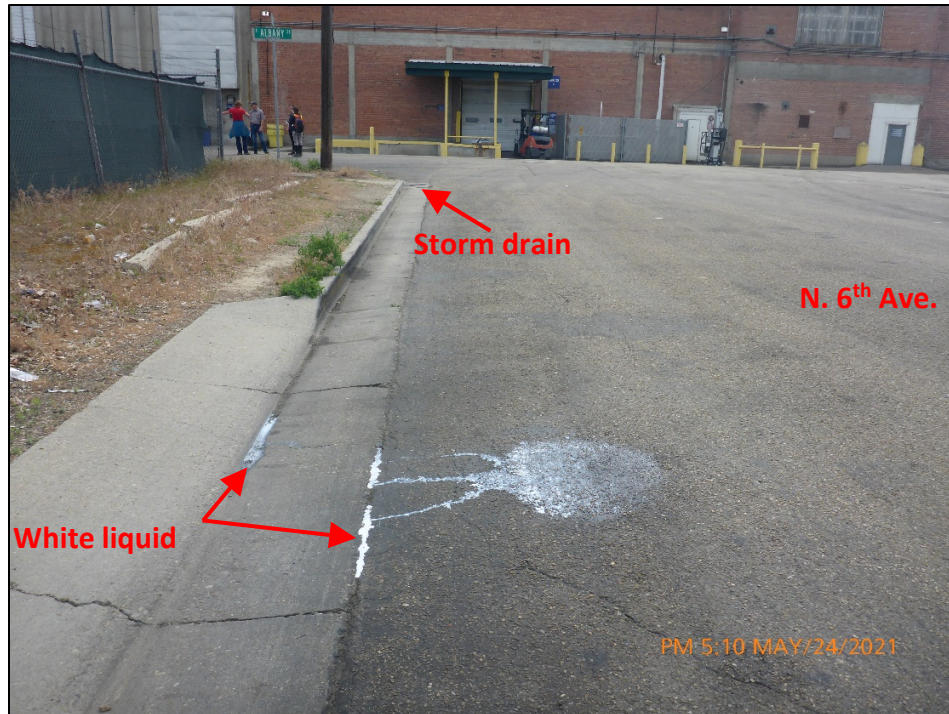
Photograph 23. View, facing southwest, of a white liquid in the gutter line of N. 6 th Ave., upgradient of the storm drain inlet at the intersection of Albany St. and N. 6 th Ave., shown in Photographs 19, 20, and 22. A milk tanker truck shown in Photo 18 is parked at this location.
