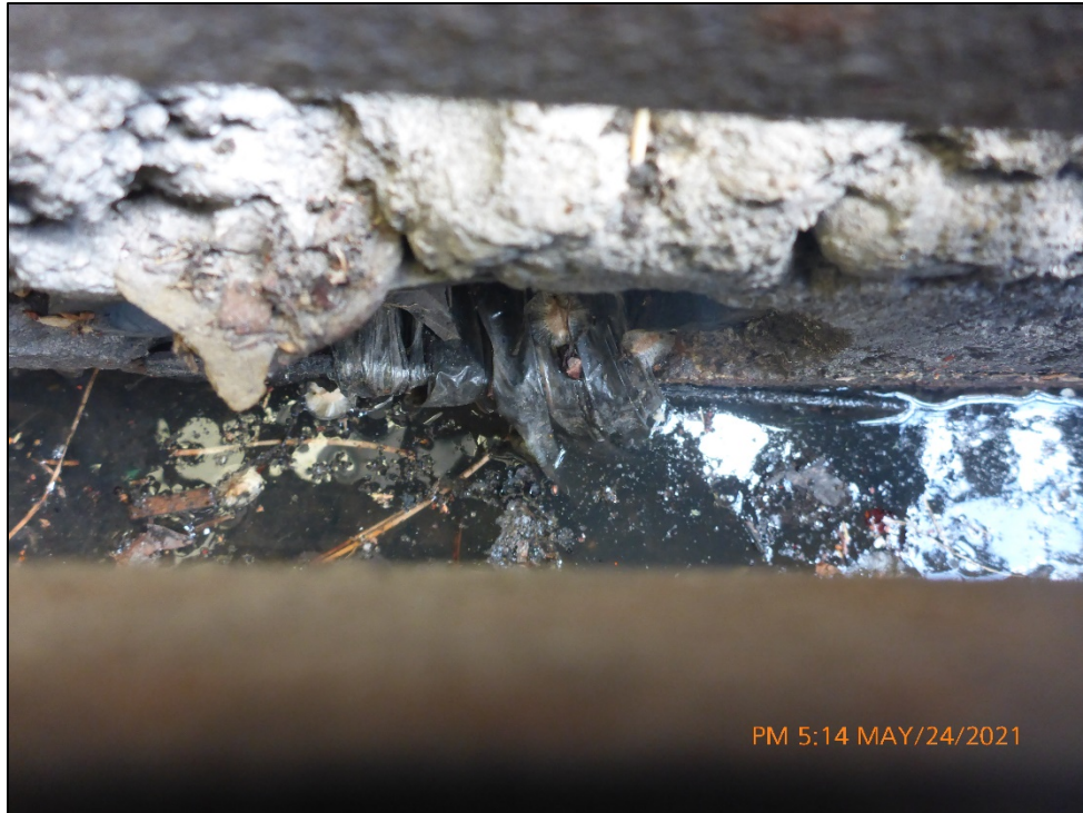
Photograph 9. View of the outlet pipe of the loading bay storm drain (Outfall 002 sample point).
