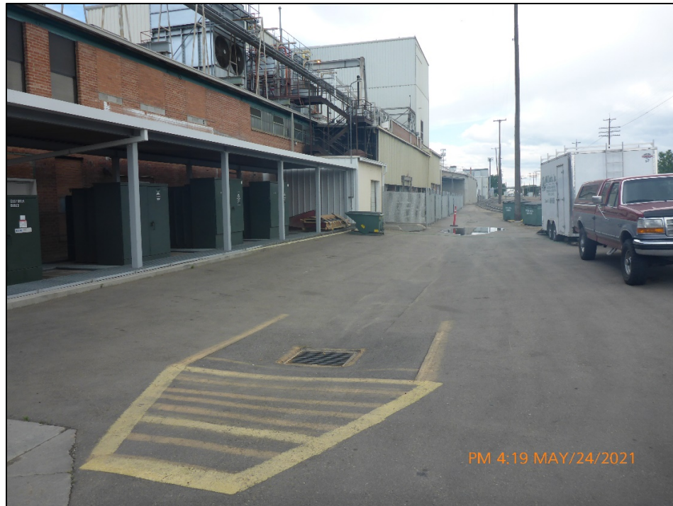
Photograph 17. View, facing southeast, of multiple storm drains along the southwestern side of the main production building that receive stormwater runoff and convey it to the Facility's wastewater treatment system. These are not identified on the SWPPP site maps.
