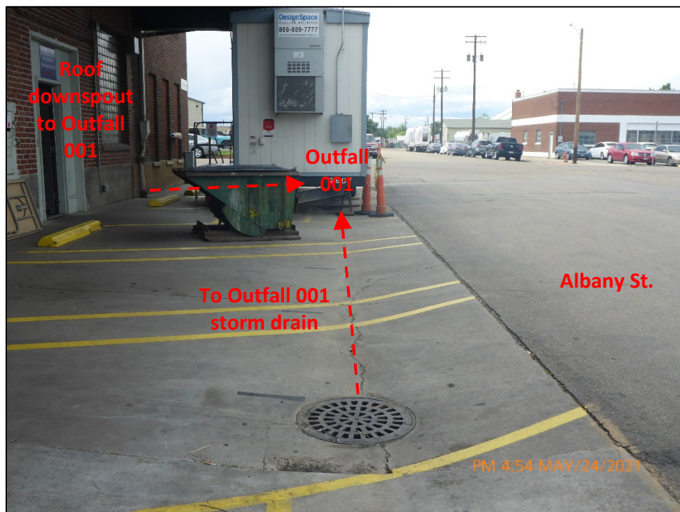
Photograph 4. View of a storm drain located southeast of Outfall 001 which receives stormwater runoff from the Facility and Albany St. This storm drain flows to Outfall 001 via the PVC pipe where Outfall 001 samples are collected.
