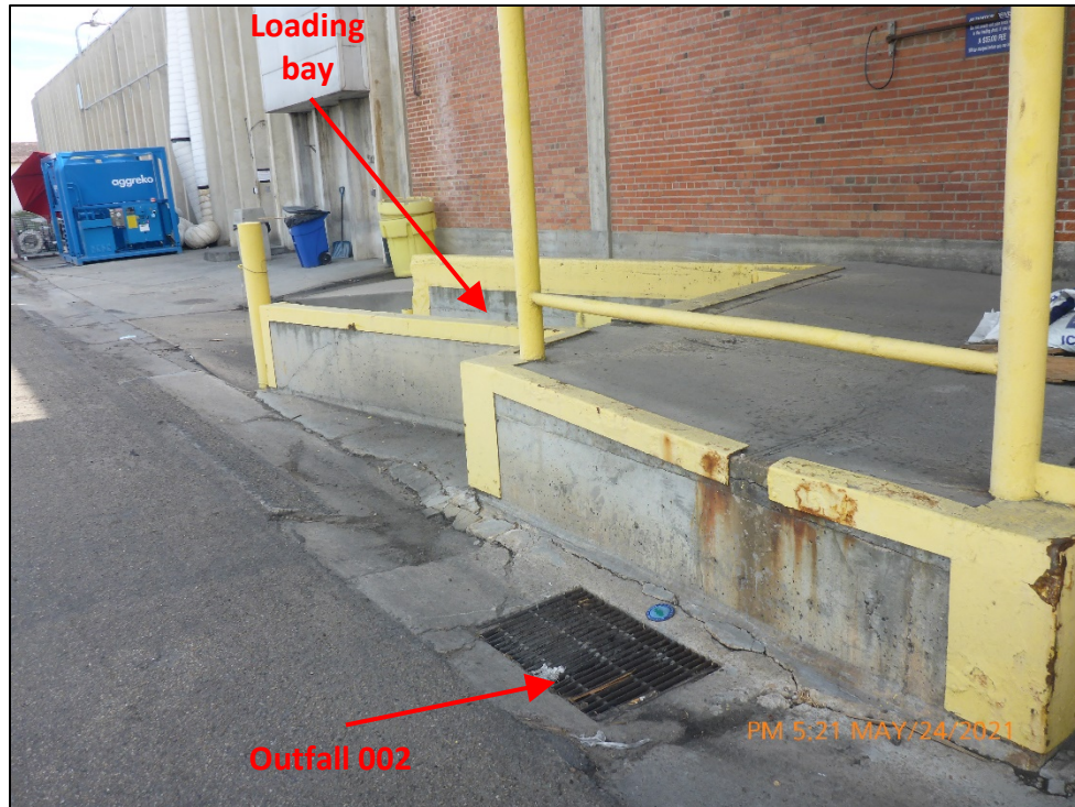
Photograph 5. View of Outfall 002. A storm drain located in the loading bay in the background is the Facility's sample point for Outfall 002, shown in Photographs 7 through 9.
