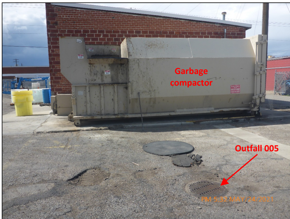
Photograph 10. View of Outfall 005 located adjacent to the garbage compactor in the eastern parcel of the Facility. Note the rubber mat is used as a storm drain cover when the compactor is emptied.
