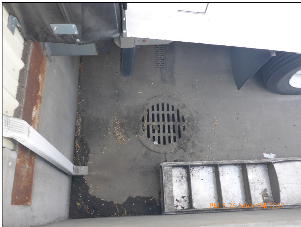
Photograph 16. View of the storm drain in the loading bay which flows to the Facility's gravel infiltration bed, as shown in Photograph 15.
