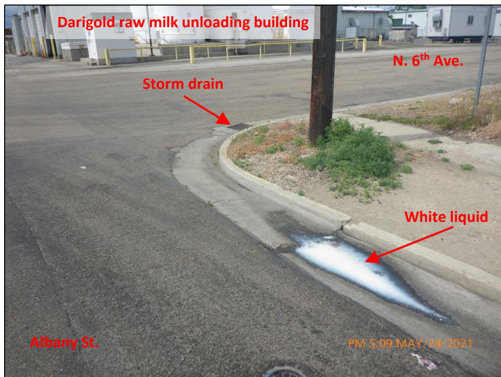
Photograph 22. Additional view, facing northwest, of white liquid in gutter line of Albany St., upgradient of the storm drain at Albany St. and N. 6 th Ave, shown in Photographs 19 through 21.
