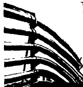
The inherent resistance of Transite Conduit to the corrosive action of many chemicals, smoke fumes and other corrosive atmospheric gases is the ideal duct for exposed runs.
