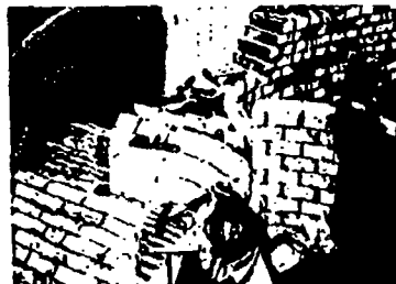
SIL-O-CEL Insulating Brick being installed with Support Brick (see page 6) in the combustion chamber of a Hot Blast Stove.
