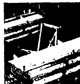
The high heat dissipation and permanence of Transite Korduct make it the desirable duct to use for steel power cables.
