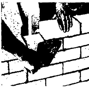
Setting Fire Brick with J-M Mortar creates a light, strong, well-protected refractory wall.
