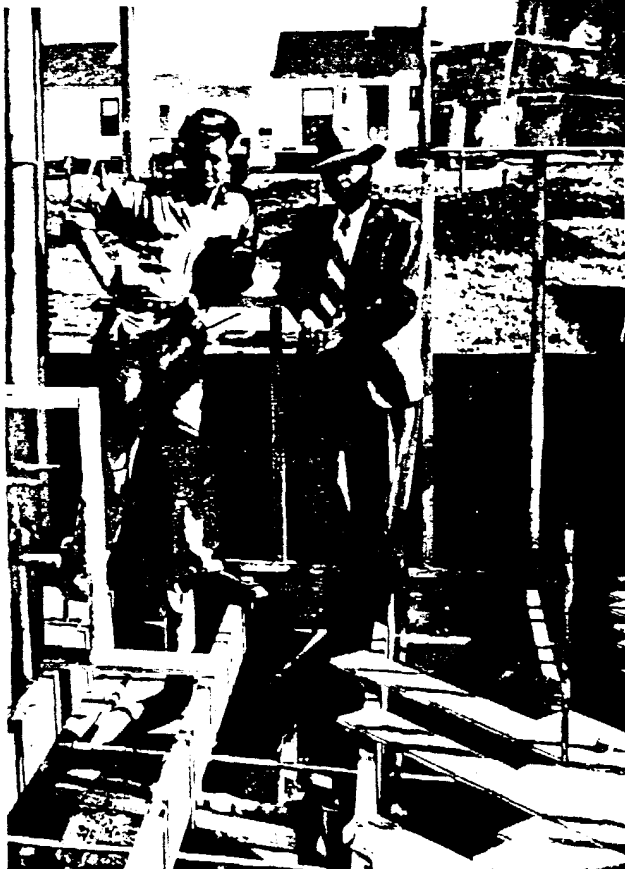
Shop fabricated standardized units of plumbing rough work ready for speedy assembly in buildings of a 125-unit housing project.
