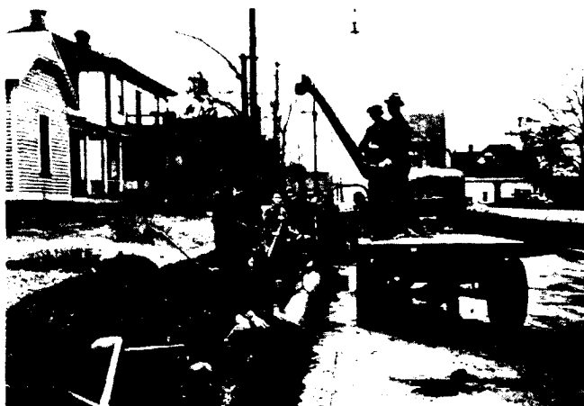
Lowering a cast-iron water main into place by derrick.
