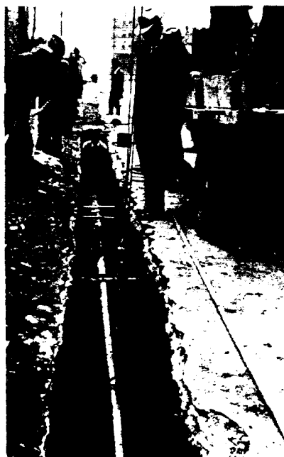
Pouring the calking lead for a cast-iron joint.
