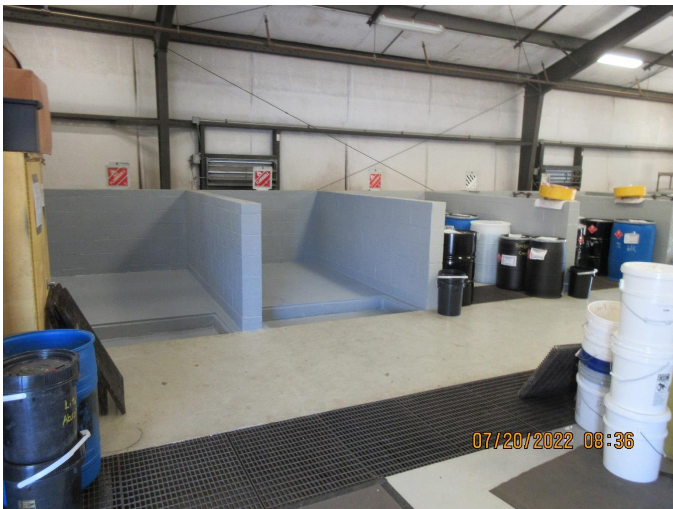
Photo 2 – Building 531 (Bays 1 & 2 on left)
