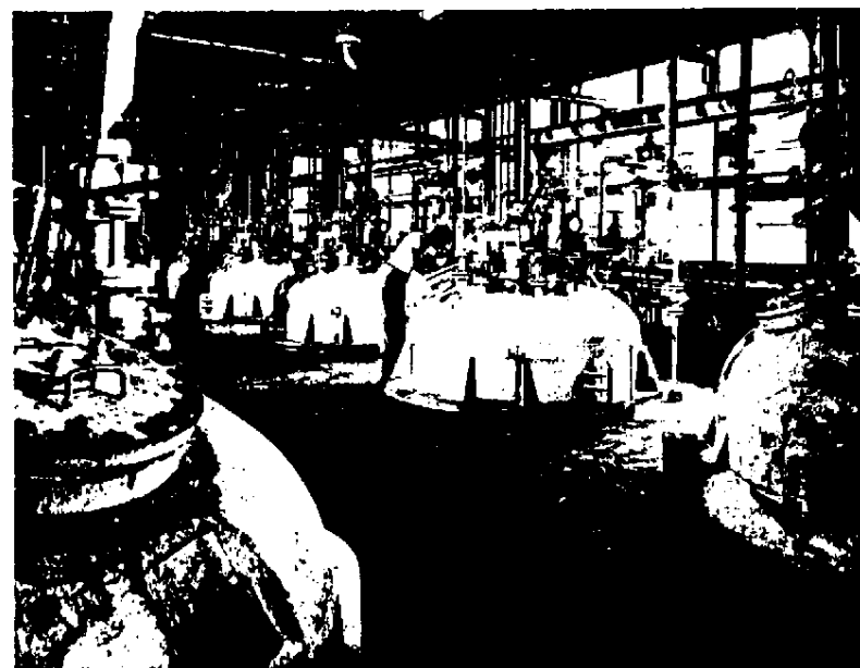
Fig 2.—Charging floor of PVC production plant showing top portion of reactors.
