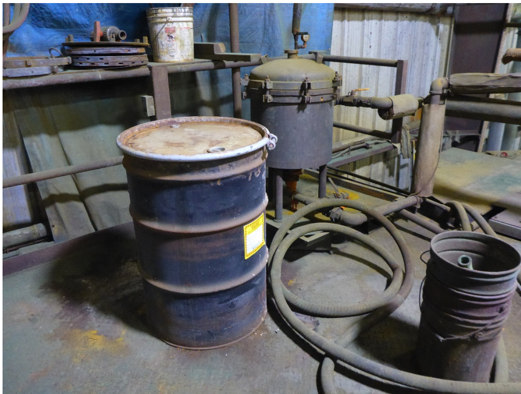
Photo 5: One 55-gallon drum in the Main Plant SAA for managing hazardous waste filter cloths that are generated in the production process. The drum was closed and labeled D007 hazardous waste solids, but it was not marked with an indication of the hazards of its contents.
