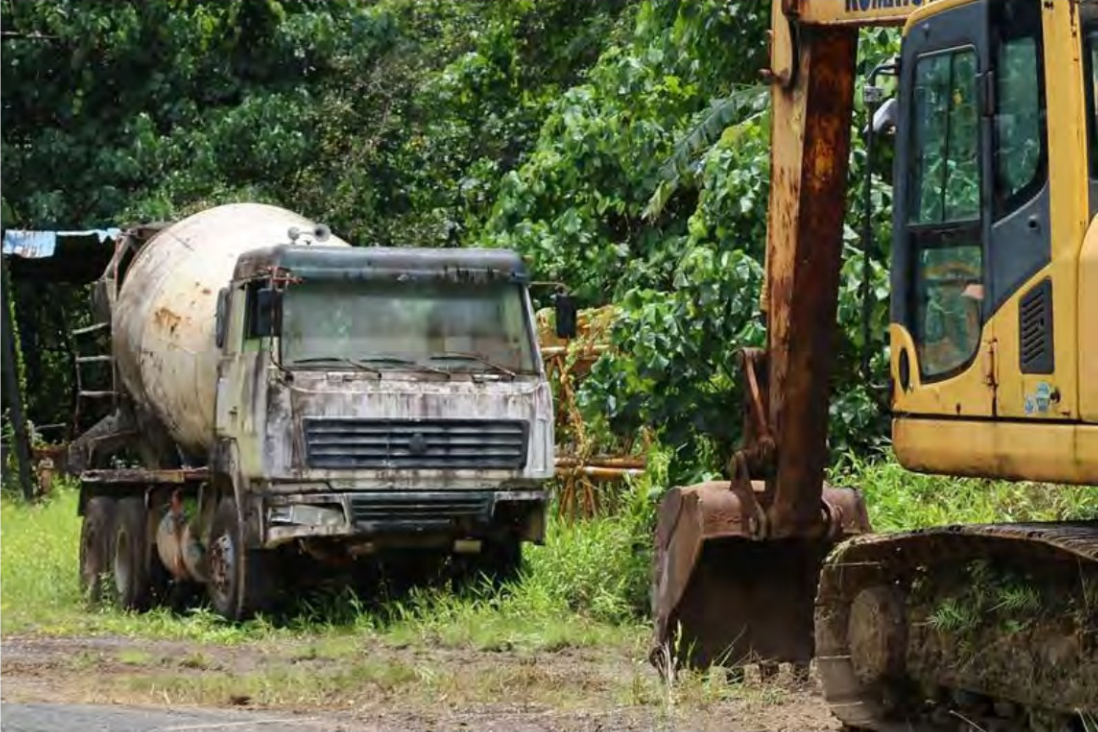
A truck and backhoe are seen at a jungle site where employees of state-owned China Railway Construction Corp. apparently live after completing a road paving project in 2021 on Pohnpei island in the Federated States of Micronesia, Aug. 20, 2023.[Stephen Wright/BenarNews] The road is one of the many Chinese projects on Pohnpei and other islands in Micronesia, a nation of some 100,000 people located between the Philippines and Hawaii that has decades-long ties with the United States.
