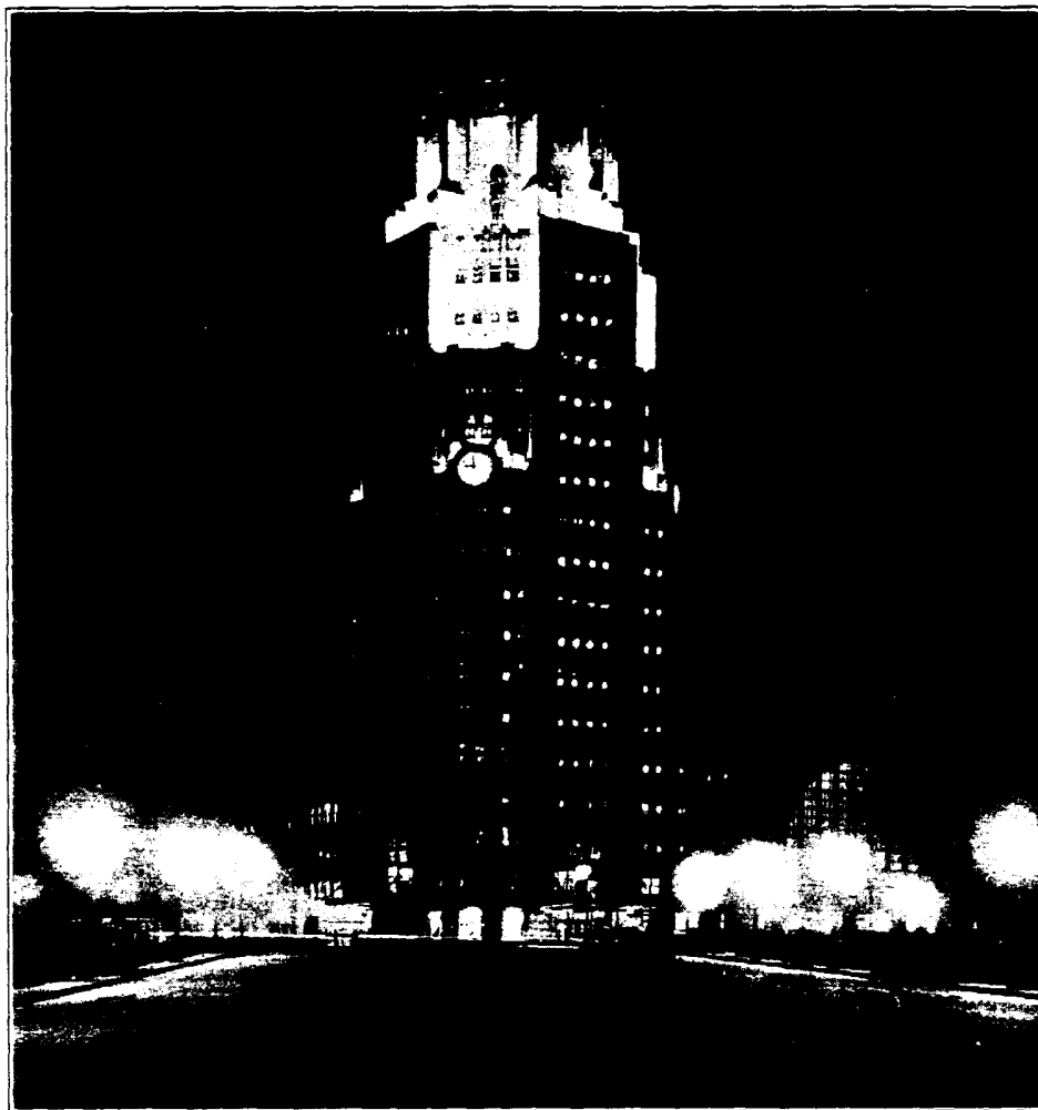
THE BUFFALO TERMINAL OF THE NEW YORK CENTRAL RAILROAD RESTS ON LEAD ANTI-VIBRATION MATTRESSES
