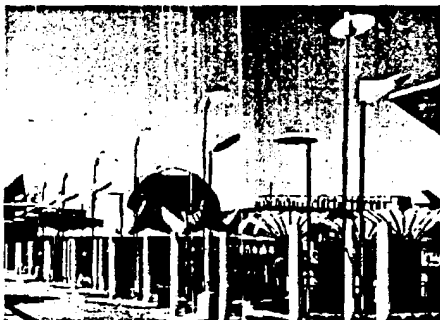
MORE THAN 2,000 Expo 67 street lighting fixtures are made of Glidden's polyester resins reinforced with fiberglass.
