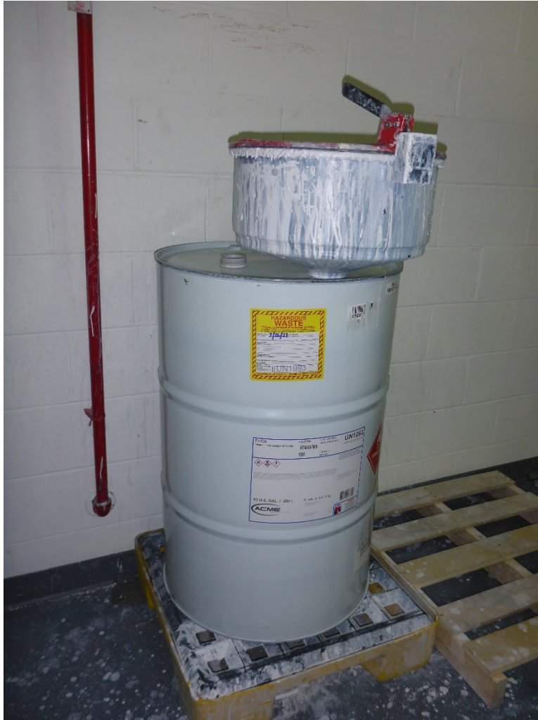
Photo 19: One 55-gallon drum located in the second solvent paint spray line SAA. The drum is located on a secondary containment pallet next to the process line. D001 / F003 / F005 hazardous waste flammable liquid (toluene / acetone) that is generated as excess paint and overspray in the solvent paint spray line is poured from the 5-gallon buckets staged at the spray line into this 55-gallon drum. The drum is closed with a latched funnel in the bung. It is labeled as D001 / F003 / F005 hazardous waste flammable liquid (toluene / acetone) and it is identified with a flammable liquid DOT hazard placard.
