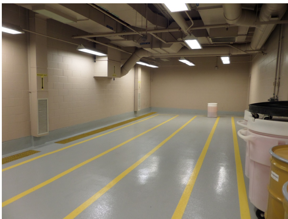
Photograph 16: Partial view of the Flammables Storage Room 115.
