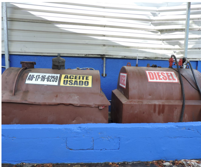
Picture 29 - DCN RECYCLING, CORP. - As observed, the Fuel and Used Oil Storage Area consisted of a metal shed with a ceiling and a secondary containment system and housed two (2) 500-gallon above ground-doble wall tanks to store used oils and diesel clearly labeled.
