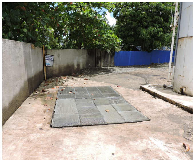
Picture 26 - DCN RECYCLING, CORP. - At the Ferrous Metal Collection Areas, there was one water tower and seep collection sump to control and manage stormwater run-on and run-off of the property. The water tower was out of service and the sump was fully filled with sediments and heavily impacted with used oils.
