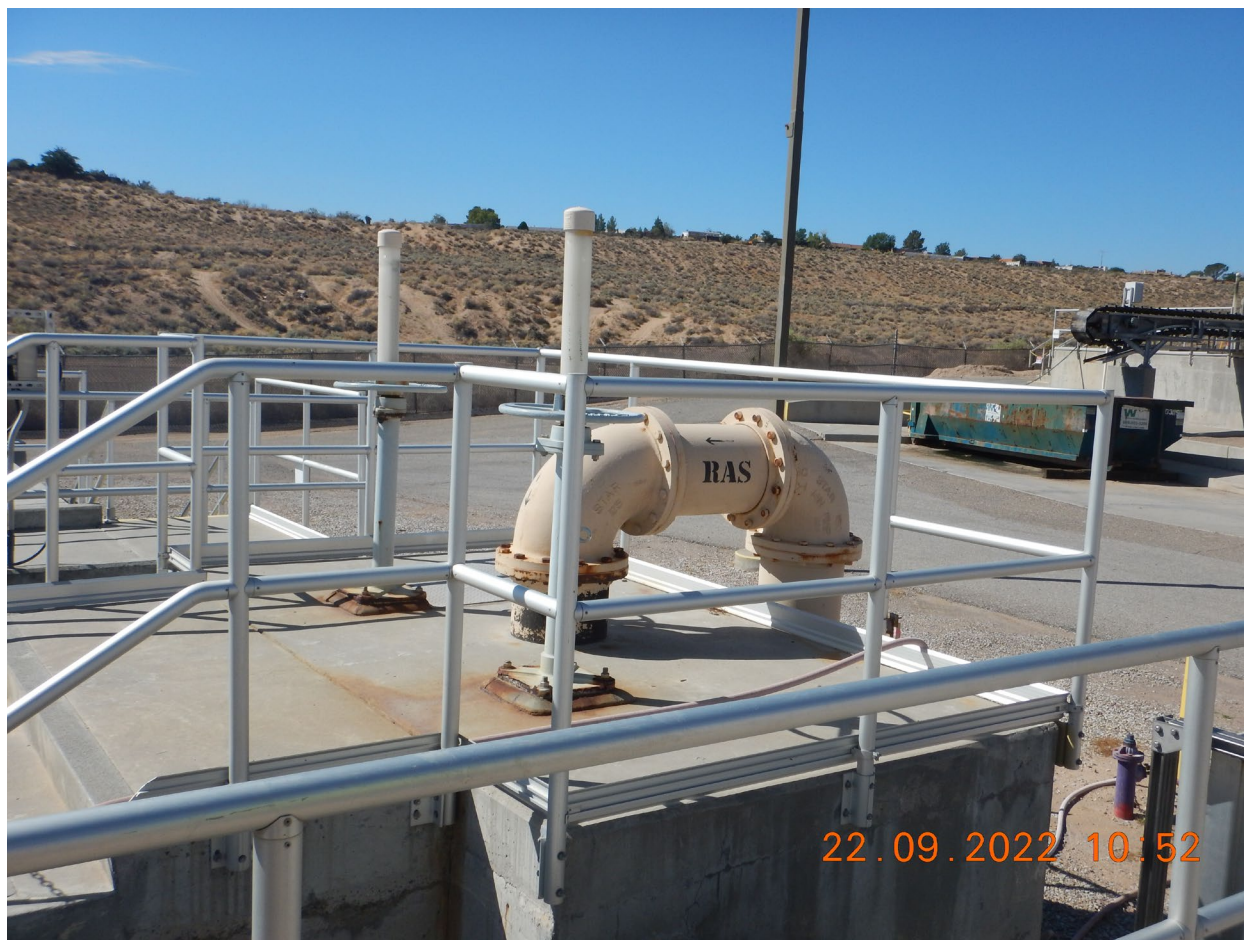
View of a spitter box looking approximately Southwest. (DSCN2330). Photographed by D. Esparza
