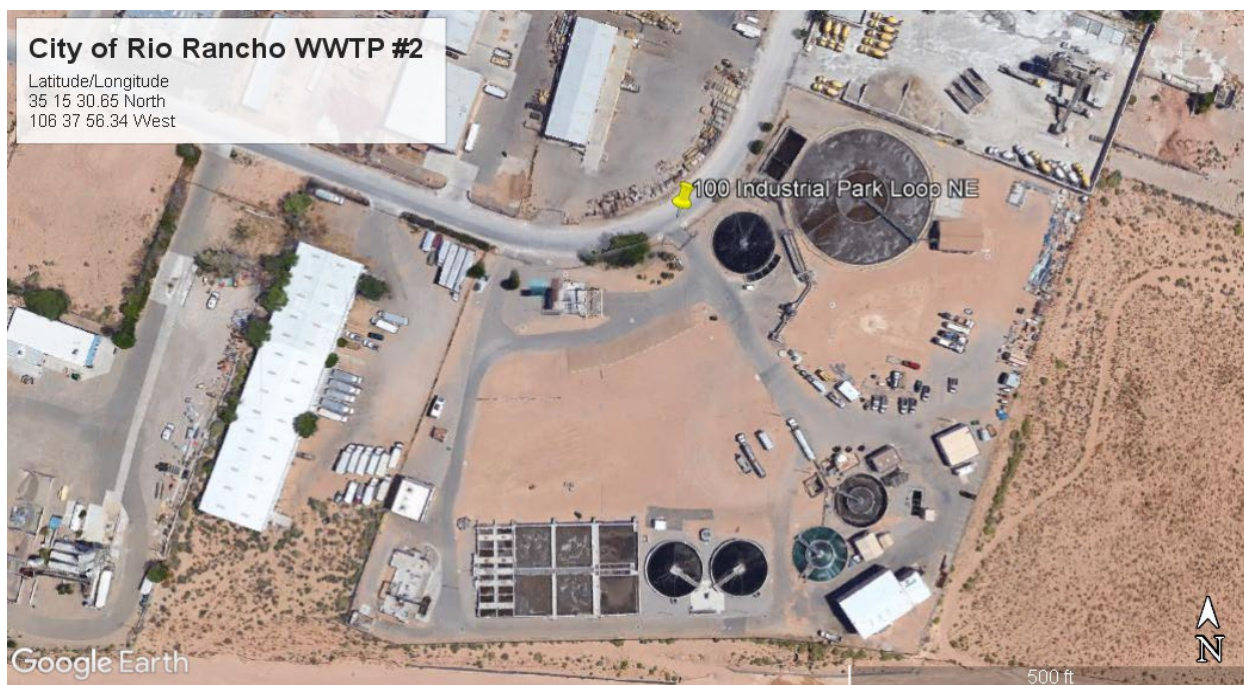
Aerial Image 1: Overall view of the City of Rio Rancho's Wastewater Treatment Plant #2. Aerial from Google Earth maps.
