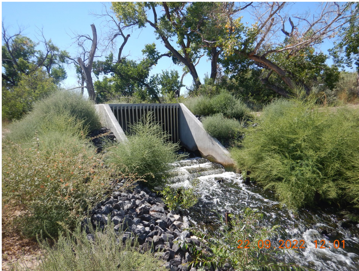
View of the new Outfall 001 discharge point. This new structure is located approximately 50-feet West of the original discharge point. (DSCN2334). Photographed by D. Esparza
