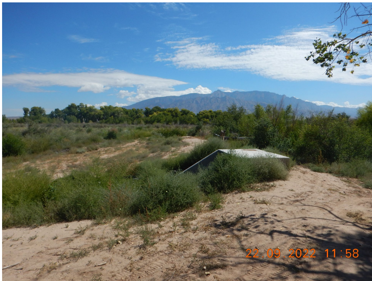
Overall view of the realigned Outfall 001 looking approximately Northeast towards the Rio Grande. (DSCN2332) Photographed by D. Esparza
