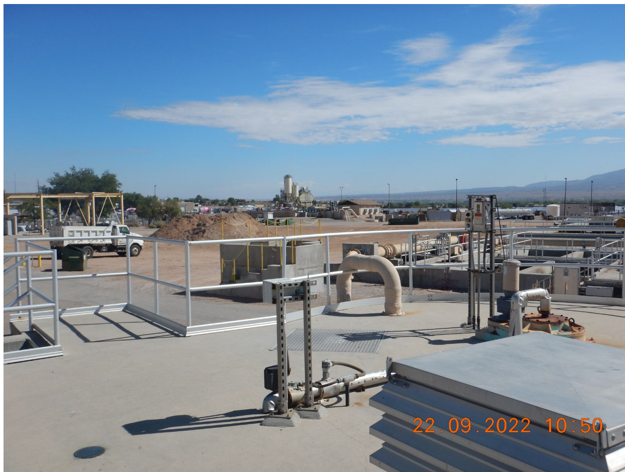
Overall view of the Rio Rancho WWTP #2 facility site looking approximately Northeast. (DSCN2329). Photographed by D. Esparza
