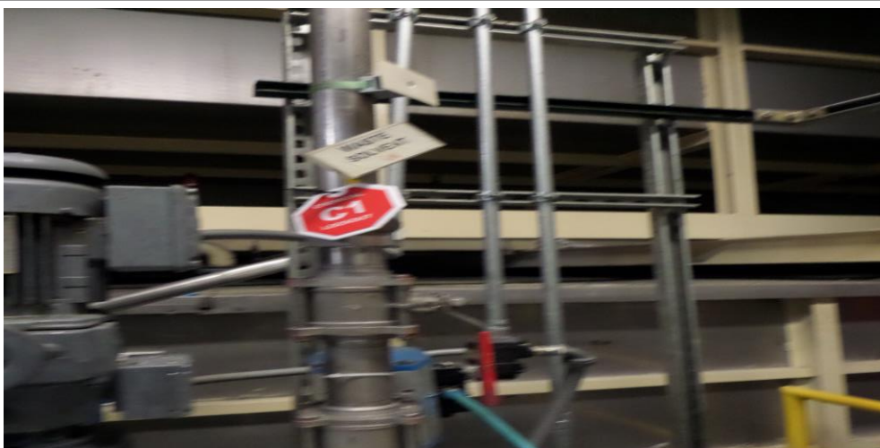
Hyundai. Kettle Purge Line 1 Area. Inspectors observed red octagonal shaped lockout tags and yellow diamond shaped tags designated with the letters C, P, E or RC and followed by a number (1, 2, or 3) secured by plastic cable ties to the tanks and the tank's ancillary equipment (valves, pumps, flanges, connectors, electrical and pneumatic equipment). Photograph 11 taken July 26, 2021 at 3:44 p.m.
