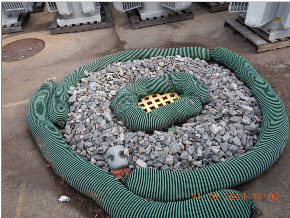
Photograph 4. DSCN0600.JPG View of a storm drain inlet in the equipment laydown area in the western portion of the Facility.
