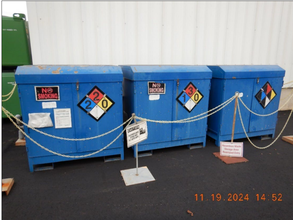
Photograph 13. DSCN0611.JPG View of the hazardous waste central accumulation area. The containers were locked, and an emergency information posting was affixed to one of the containers.
