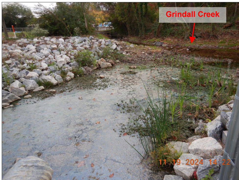
Photograph 8. DSCN0605.JPG View of Outfall 003 to Grindall Creek.
