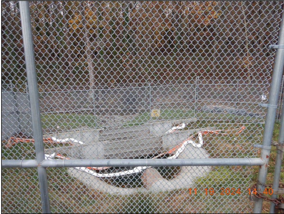
Photograph 9. DSCN0607.JPG View of Outfall 001 to Grindall Creek. The outfall structures were located inside a fence associated with construction activity.
