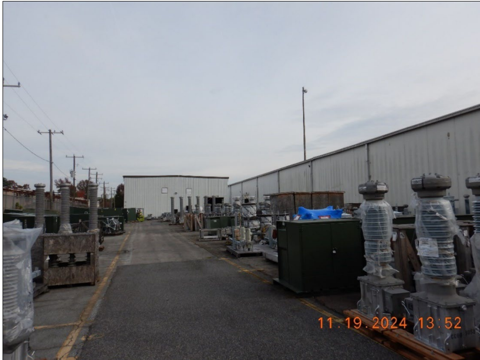
Photograph 1. DSCN0596.JPG View of the equipment laydown area in the northern portion of the Facility.
