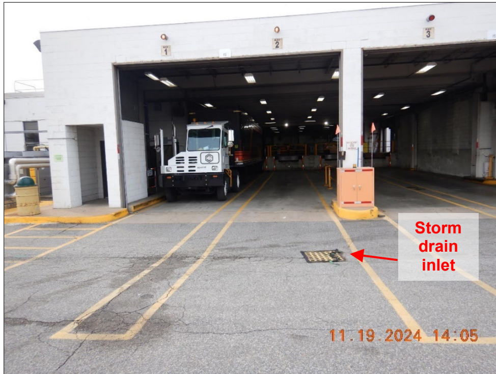
Photograph 5. DSCN0601.JPG View of the truck unloading area on the east side of the shops building. Stormwater that enters this inlet flows to the oil sensor sump system prior to being discharged via Outfall 001.
