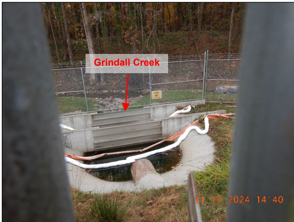
Photograph 10. DSCN0606.JPG Additional view of Outfall 001 to Grindall Creek.
