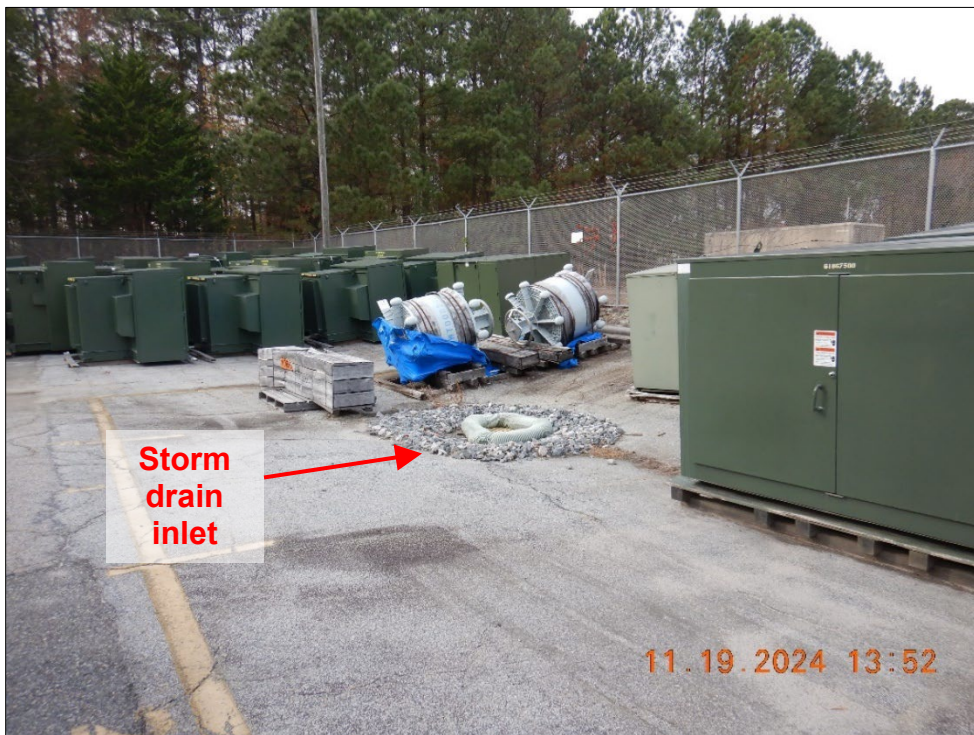
Photograph 2. DSCN0597.JPG View, facing northwest, of a storm drain inlet in the northwest corner of the Facility in the equipment laydown area.
