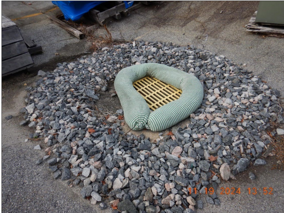
Photograph 3. DSCN0598.JPG Close-up view of the storm drain inlet shown in Photograph 2.
