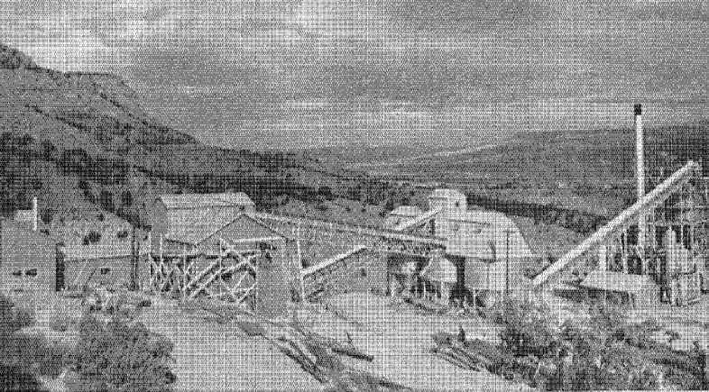
This is an overall view of the plant, near Rifle, Colorado, for heating the crushed shale to extract its oil content.
