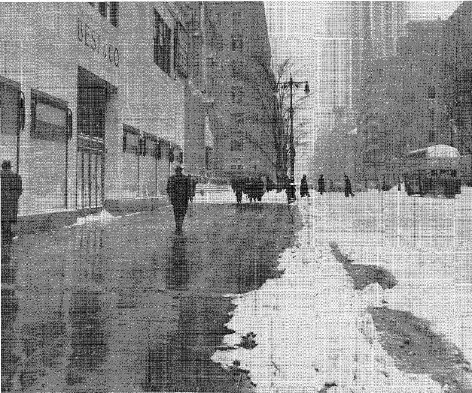
Snow didn't stay on this sidewalk during New York's blizzard of '47, for the pavement was "heated."
