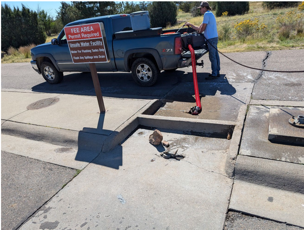
Figure 3 - Chatfield State Park - RV Dump Station
