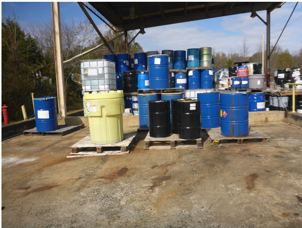
Photo 1: Six pallets, which are arranged in four rows and not stacked, in the curbed concrete pad CAA in the facility yard. (Note that the stacked containers shown behind the CAA are in the Building 19 Covered Storage Pad.)
