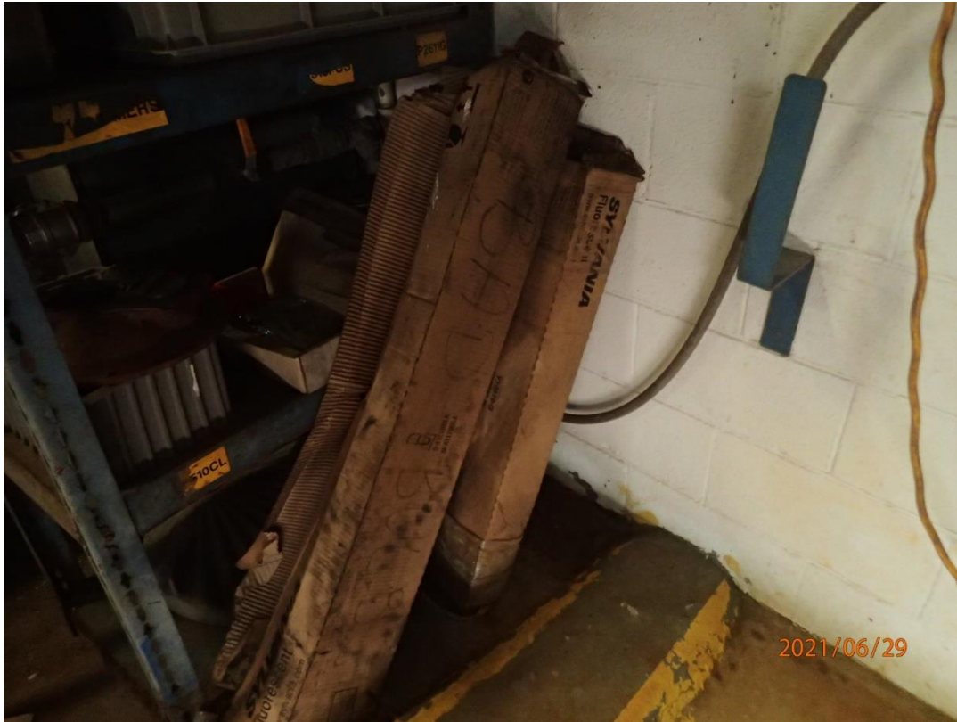
Photo 7: Two (2) boxes of fluorescent lamps labeled “Bad Bulbs” were also observed on the first floor of the WWTP.
