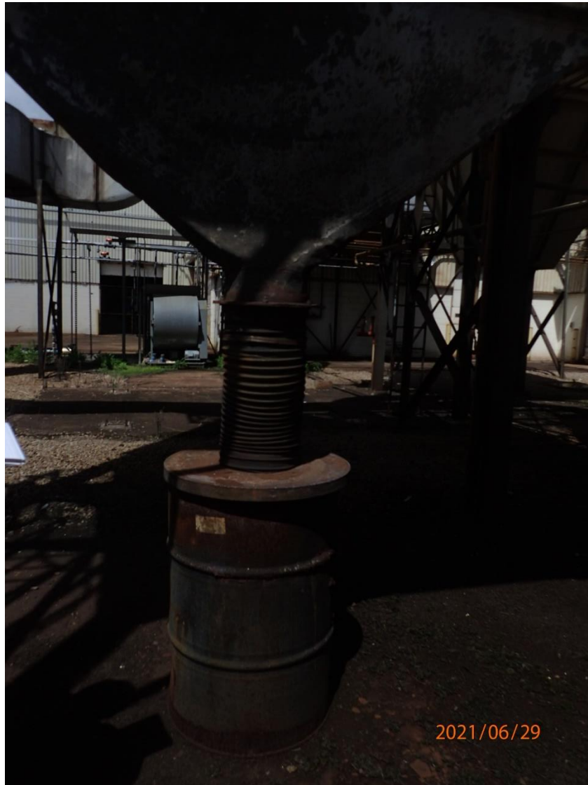
Photo 12: One of two 55-gallon containers attached to the baghouses. The container was not labeled.
