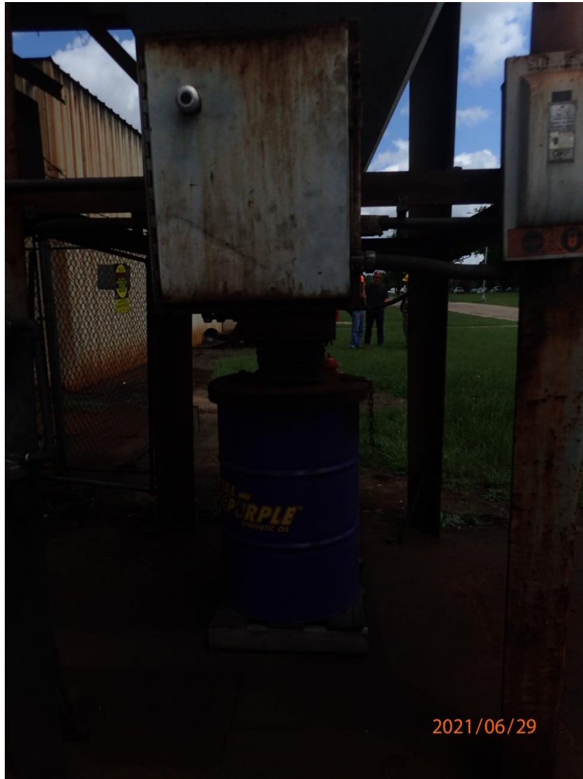
Photo 17: 55-gallon drum connected to a baghouse just outside of the Back Building, managed as non-hazardous waste
