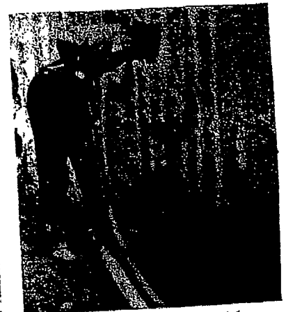
A dangerous concentration of silica dust at left, thrown off in a cloud by a pneumatic drill. On the right a new suction collector carries away all dust
