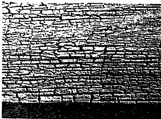
Abnormal disintegration of paint by alligatoring. In this case a pigment house paint was applied over a clear varnish used as a wood sealer in place of a paint primer.
