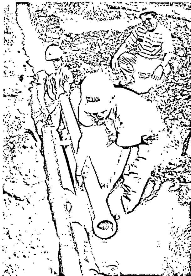
This bank of asbestos-cement pipe will ensure watertightness for electrical cables.
