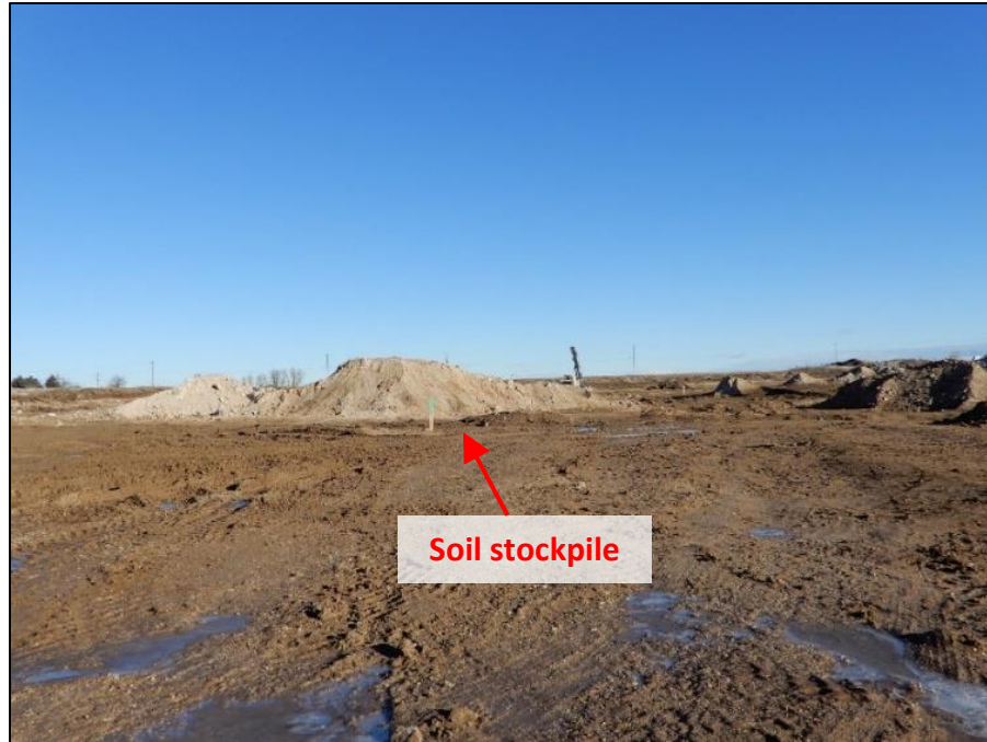
Photograph 3. View, facing north, of unstabilized soil stockpile located at the south-central area of the Site. Downgradient perimeter controls were observed.
