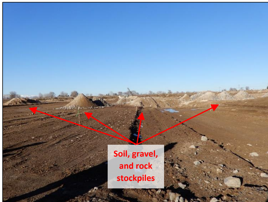
Photograph 2. View, facing west, of four locations of unstabilized soil, gravel, and rock stockpiles located at the center of the Site. Downgradient perimeter controls were observed at the Site's southern perimeter.
