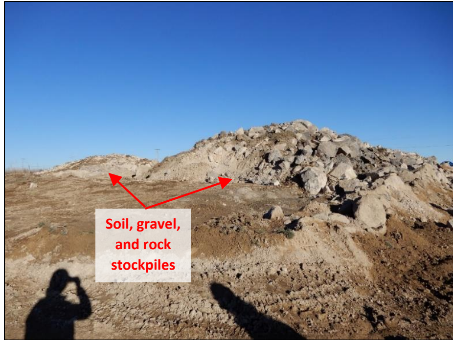
Photograph 1. View, facing west, of two unstabilized soil, gravel, and rock stockpiles located at the north-central location of the Site. Downgradient perimeter controls were observed.
