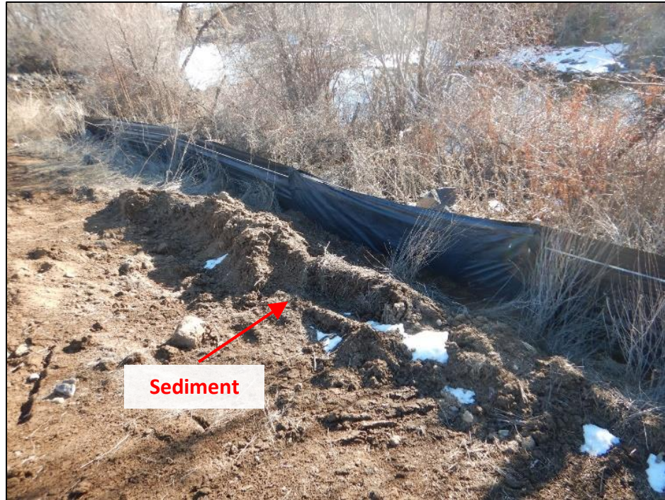
Photograph 7. View, facing southeast, of sediment that had accumulated to approximately one-half of the above-ground height of the silt fence. The sediment is located east of Photograph 5 .
