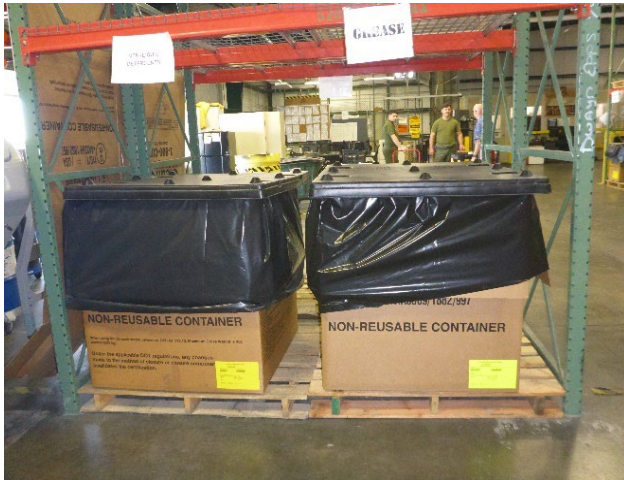
Photo 8: Bay C1 for consolidating and storing non-liquid detergents and grease in the CAA.
