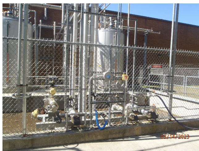
Figure 33: P3140046.JPG: Loading and unloading area
