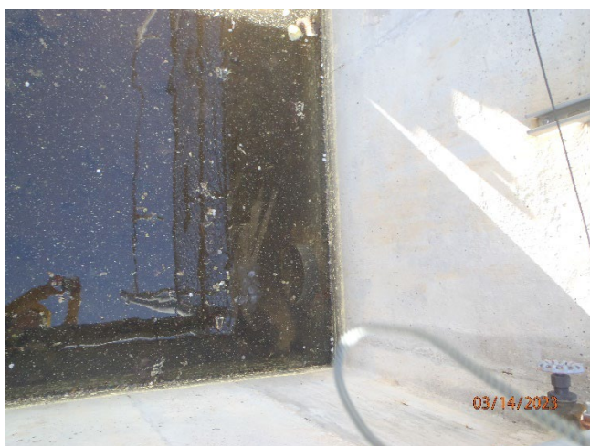
Figure 19: P3140031.JPG: Secondary Containment Pit
