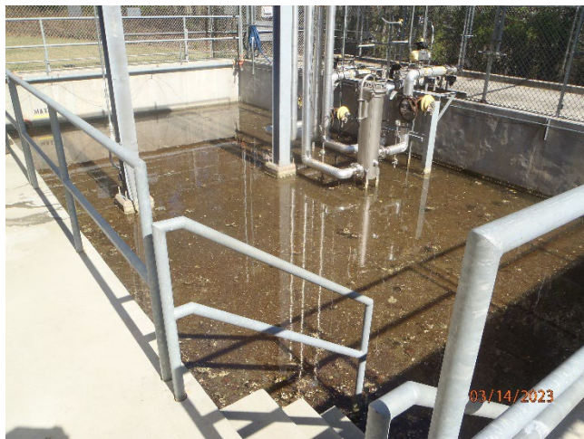
Figure 7: P3140014.JPG: Secondary Containment Pit
