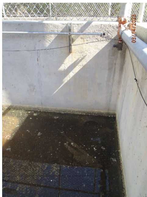
Figure 18: P3140030.JPG: Secondary Containment Pit
