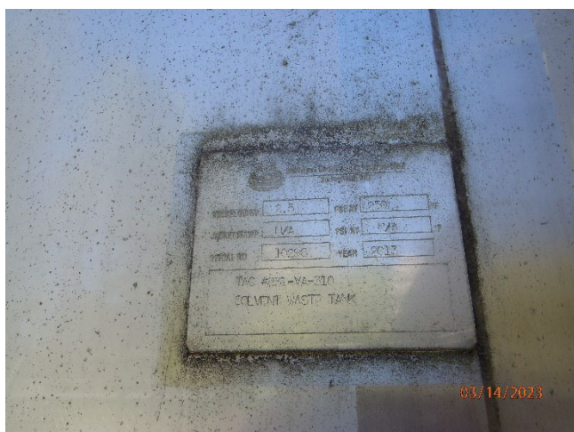
Figure 31: P3140043.JPG: Manufacturer's Plate on the Used Acetone Tank
