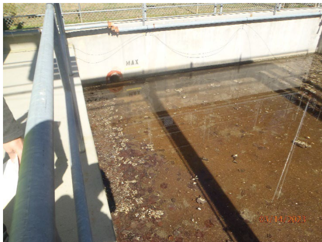
Figure 10: P3140018.JPG: Secondary Containment Pit
