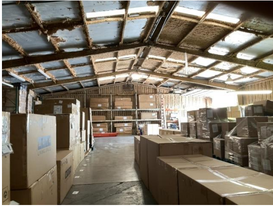
Photo 1: Building 1 Warehouse. No hazardous waste observed.
