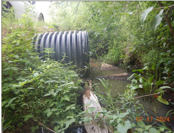
Paul Goodwin Date: 17 July 2024 Photo ID: DSCN5487.JPG Photo taken by: Laura Mathew Notes: West facing view of UNT1 and inlet of culvert 1B.
