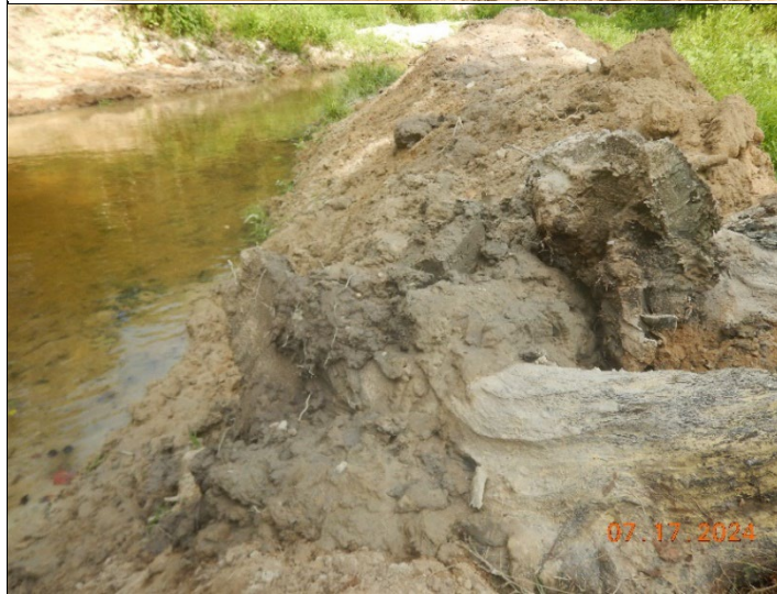
Paul Goodwin Date: 17 July 2024 Photo ID: DSCN5516.JPG Photo taken by: Laura Mathew Notes: Closeup view of the newly constructed berm.
