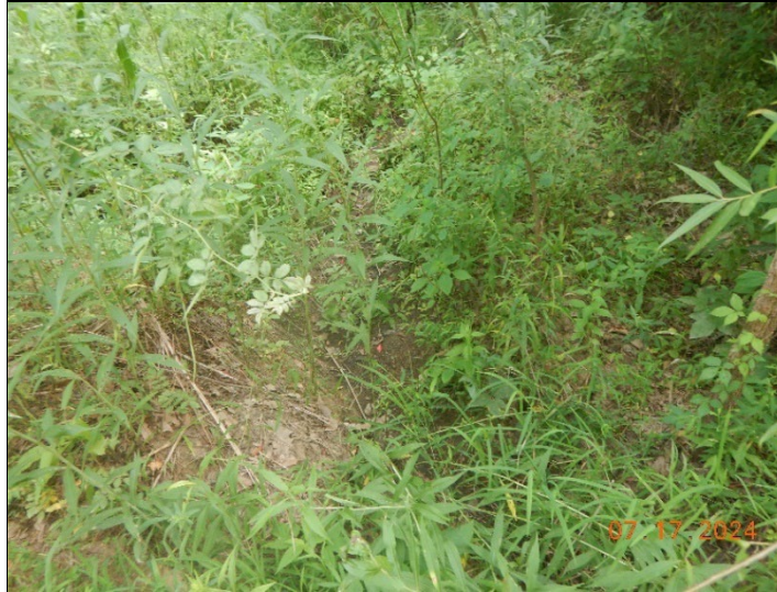
Paul Goodwin Date: 17 July 2024 Photo ID: DSCN5483.JPG Photo taken by: Laura Mathew Notes: Inlet of existing culvert 1A.
