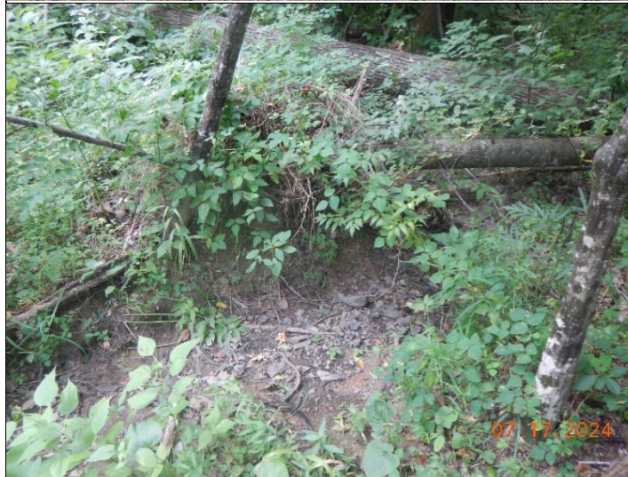
Paul Goodwin Date: 17 July 2024 Photo ID: DSCN5485.JPG Photo taken by: Laura Mathew Notes: Downstream view of culvert 1A.
