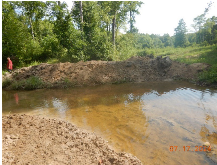
Paul Goodwin Date: 17 July 2024 Photo ID: DSCN5514.JPG Photo taken by: Laura Mathew Notes: Eastward view of the newly constructed berm.
