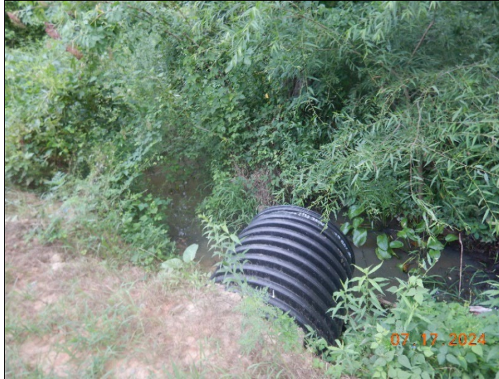
Paul Goodwin Date: 17 July 2024 Photo ID: DSCN5486.JPG Photo taken by: Laura Mathew Notes: UNT1 and inlet of existing culvert 1B.
