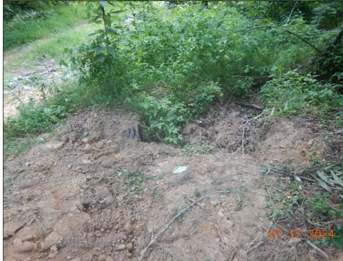
Paul Goodwin Date: 17 July 2024 Photo ID: DSCN5484.JPG Photo taken by: Laura Mathew Notes: Outlet of existing culvert 1A.
