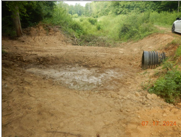
Paul Goodwin Date: 17 July 2024 Photo ID: DSCN5488.JPG Photo taken by: Laura Mathew Notes: Outlet of culvert 1B.
