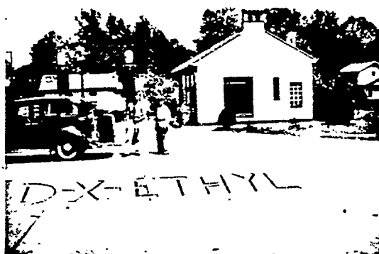
• Top: C. E. Colvin demonstrates at a MidContinent S. S. and below a typical demonstration. Harry Kuhe and H. N. Peters of Tulsa Division are first and third from left, directly above view of S. S. with three foot letters painted on drive.
