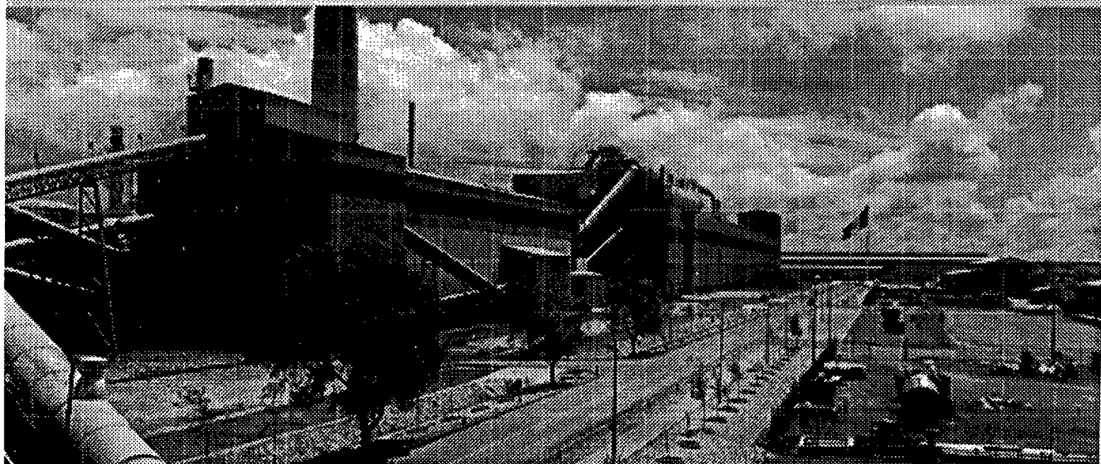
Partial view of Metallurgical Complex La Caridad, Sonora
