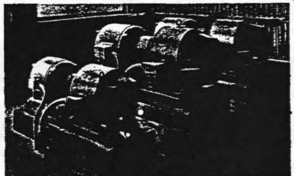
These are the motor-generator sets that supply synchronous motor excitation.
