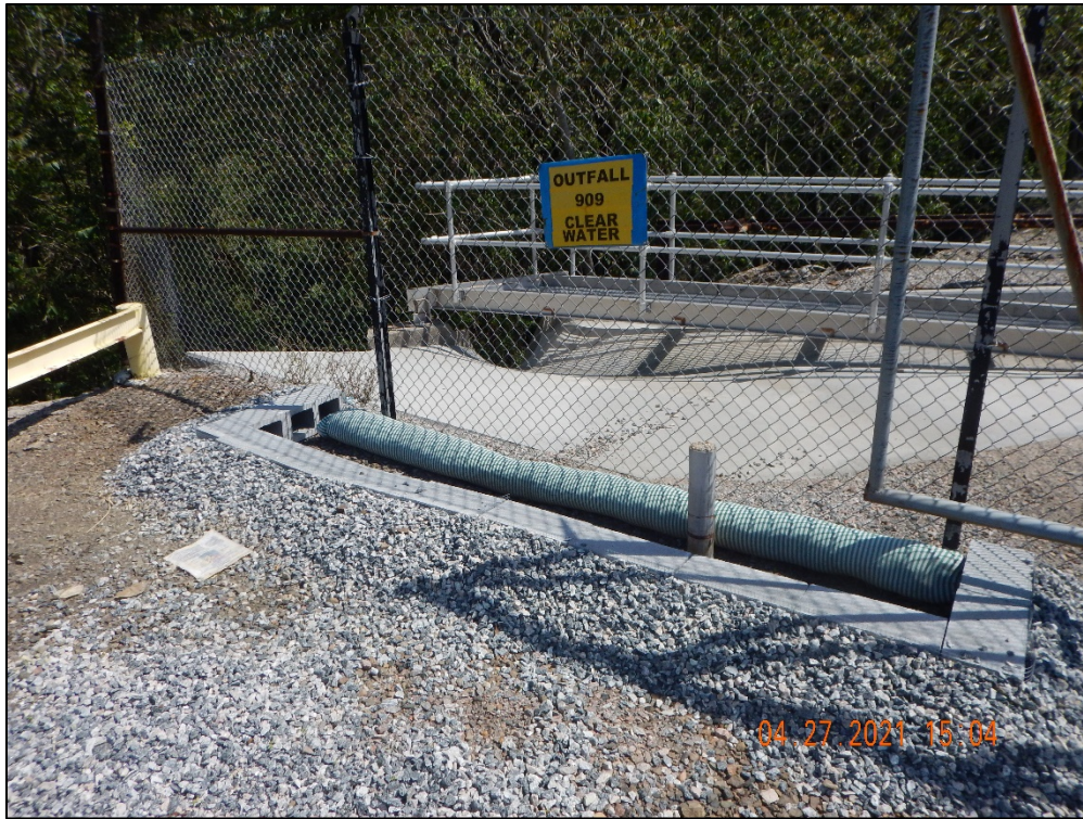
DSCN2393. View, facing south, of Outfall 909 to Gravelly Run. Outfall 909 receives stormwater from a single stormwater inlet in a small parking lot.
