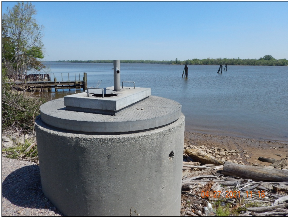
DSCN2340. View, facing east, of the final manhole upgradient of Outfall 906. Facility representatives stated that the actual outfall was currently submerged in the James River.
