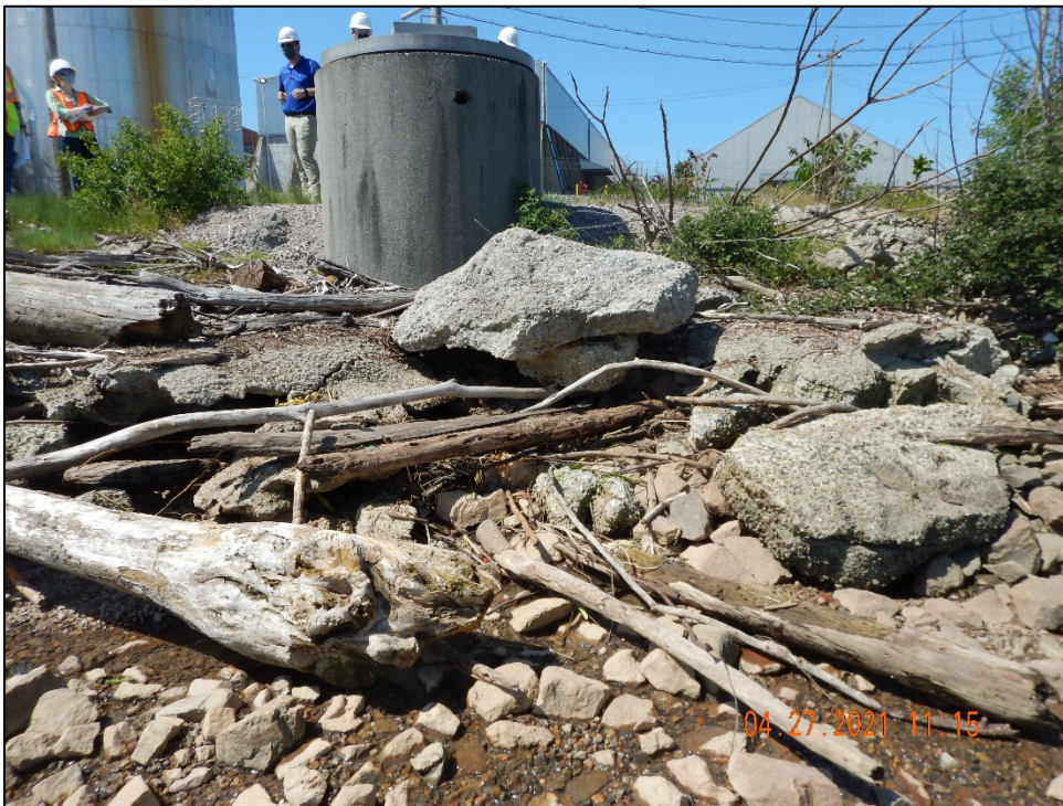
DSCN2339. View, facing west, of the final manhole upgradient of Outfall 906. The EPA Inspection Team observed a small amount of water draining from the manhole.
