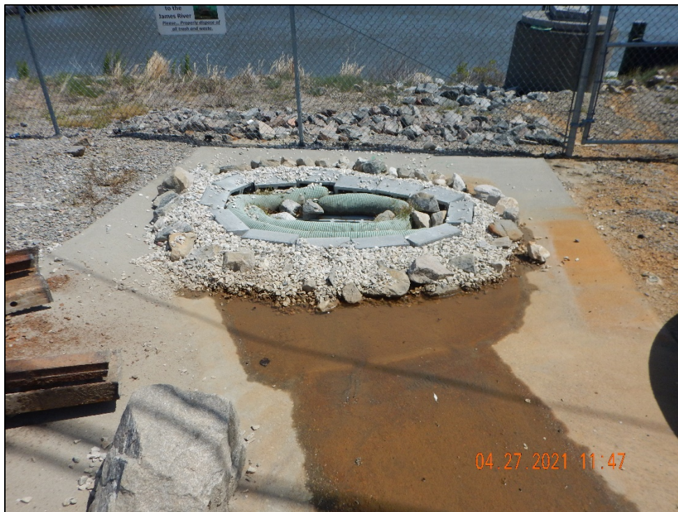
DSCN2355. View, facing east, of the third sampling point upgradient of Outfall 904. The EPA Inspection Team observed dry-weather flow to this inlet.
