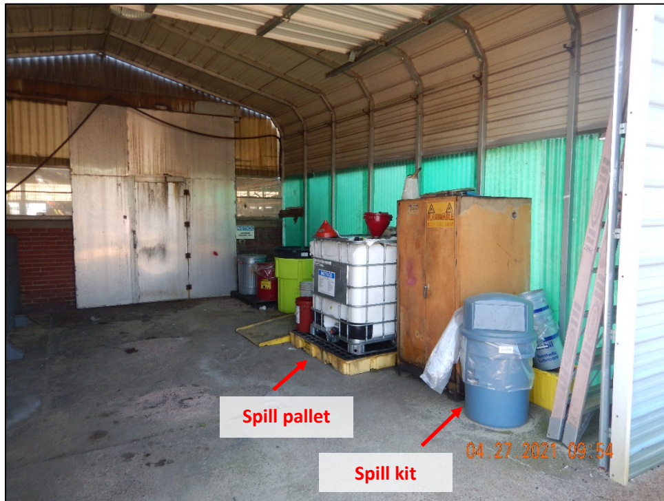
DSCN2306. View inside the covered drum shed in the North Maintenance Shop. Note the used oil tote on a spill pallet and the presence of a spill kit.
