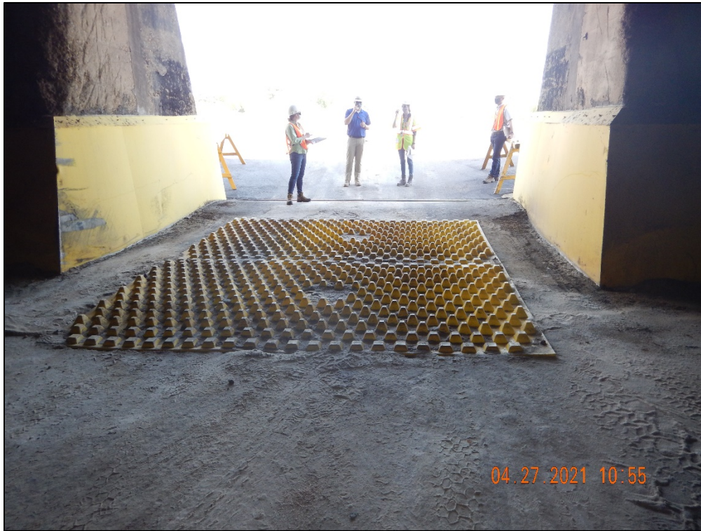
DSCN2331. View, facing north, of the yellow foreign object debris system in the entryway to the fertilizer warehouse. It is used to reduce the fertilizer track-out on dump truck tires.
