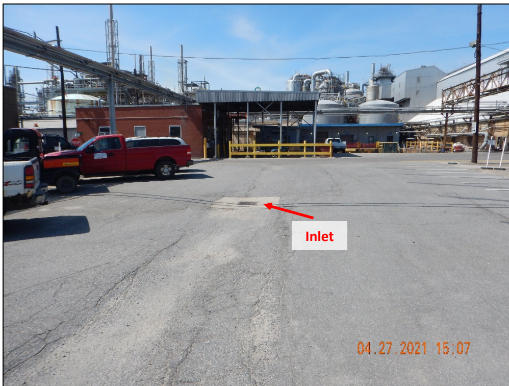
DSCN2394. View, facing north, of the single inlet draining to Outfall 909.
