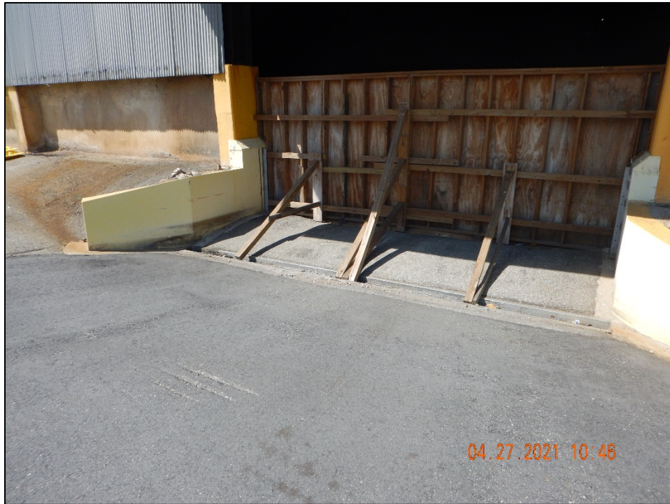
DSCN2328. View, facing west, of the entryway to the northernmost fertilizer warehouse. Facility representatives stated that this warehouse was no longer used.
