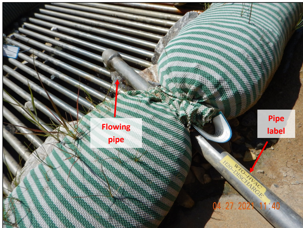
DSCN2349. View of the small pipe labelled “WTO-HVAC H2O-DISCHARGE” flowing into the inlet upgradient of Outfall 905.
