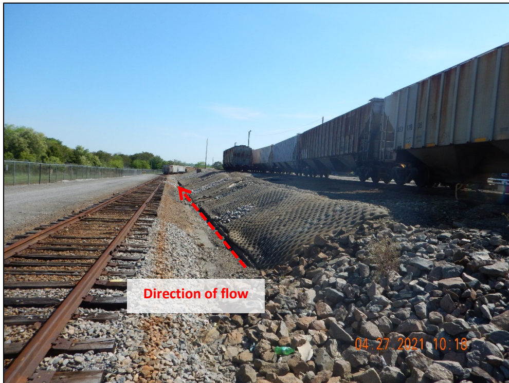
DSCN2317. View, facing east, of the slope between the rail tracks and the north perimeter fence. Note the concrete stabilization on the slope.
