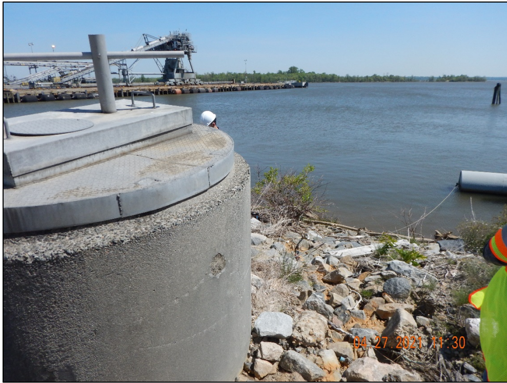
DSCN2345. View, facing northeast, of the final manhole upgradient of Outfall 904. Facility representatives stated the actual outfall was submerged in the James River.
