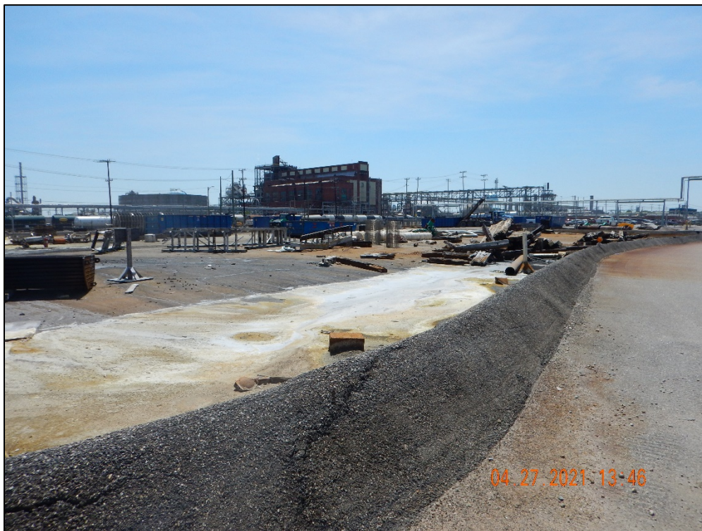
DSCN2369. View, facing southwest, of the bermed equipment lay-down area. Facility representatives stated this area drains to the process waste sewer system.
