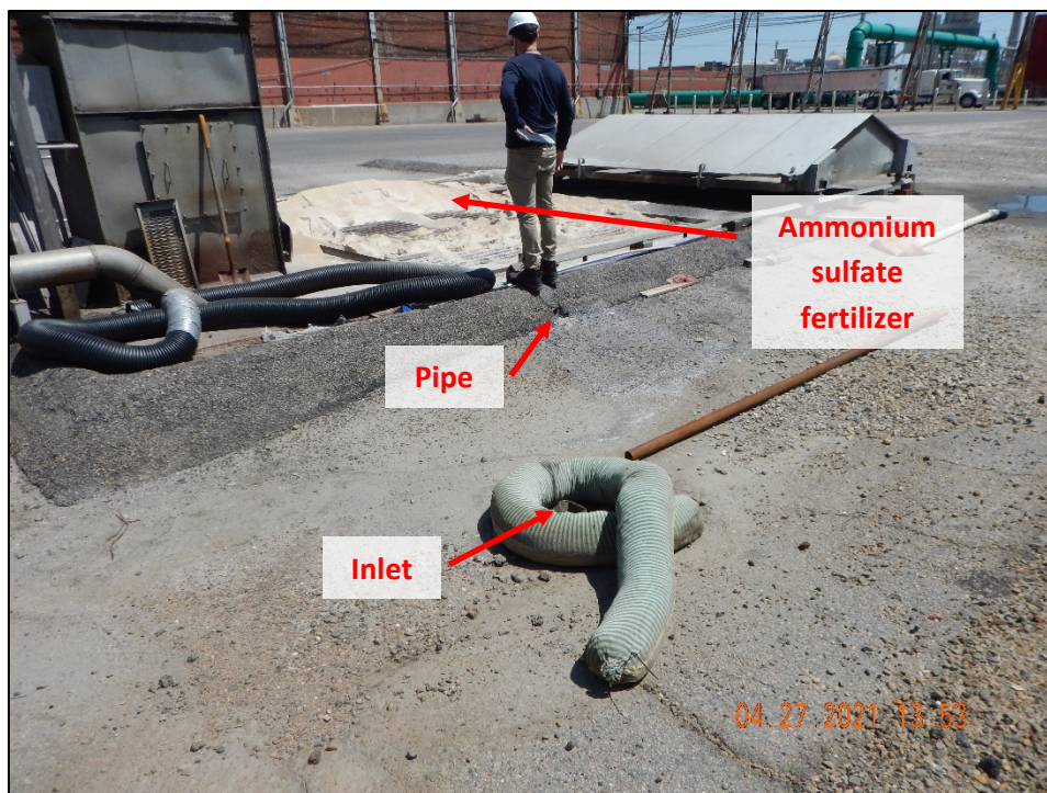
DSCN2373. View, facing southeast, of another stormwater inlet located approximately 10 feet from the ammonium sulfate fertilizer pit.
