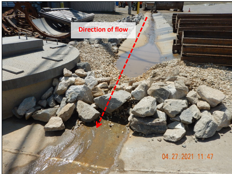
DSCN2356. View, facing southwest, of a ditch with dry-weather flow running to the inlet from DSCN 2355.
