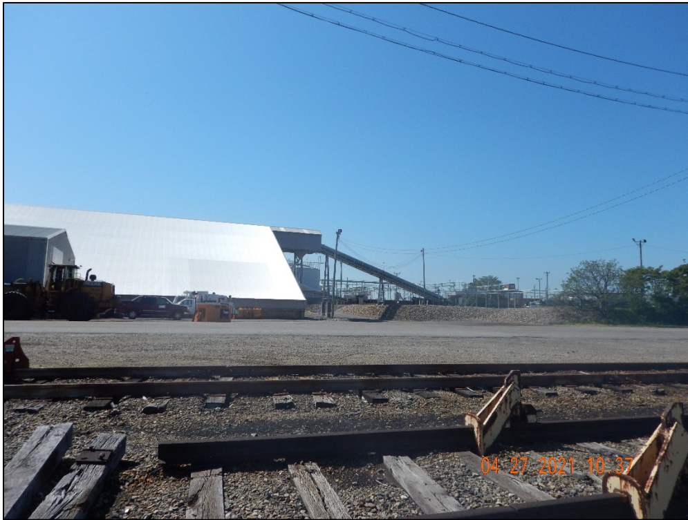
DSCN2324. View, facing south, of one of the two main ammonium sulfate storage warehouses in the northeast corner of the Facility. The second warehouse is behind the large white building.
