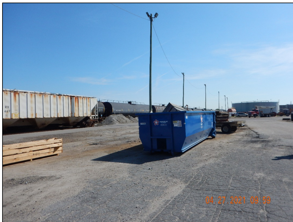
DSCN2308. View, facing east, of an uncovered scrap metal dumpster in the Outfall 912 drainage area.
