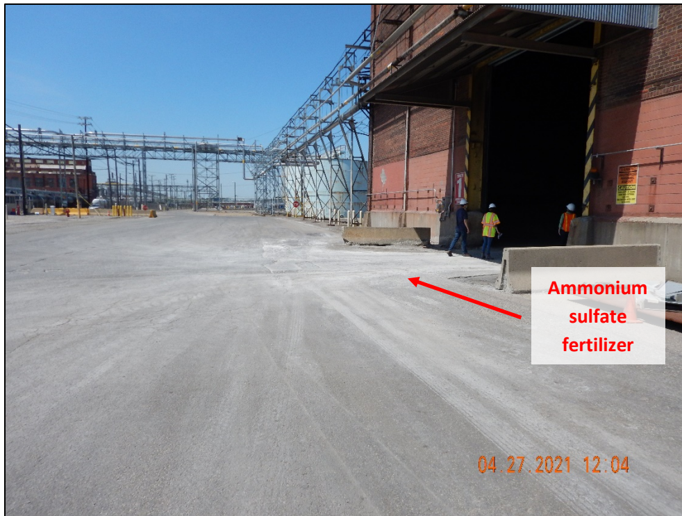
DSCN2365. View, facing west, of ammonium sulfate fertilizer track-out in front of a storage warehouse in the Outfall 904 drainage area.
