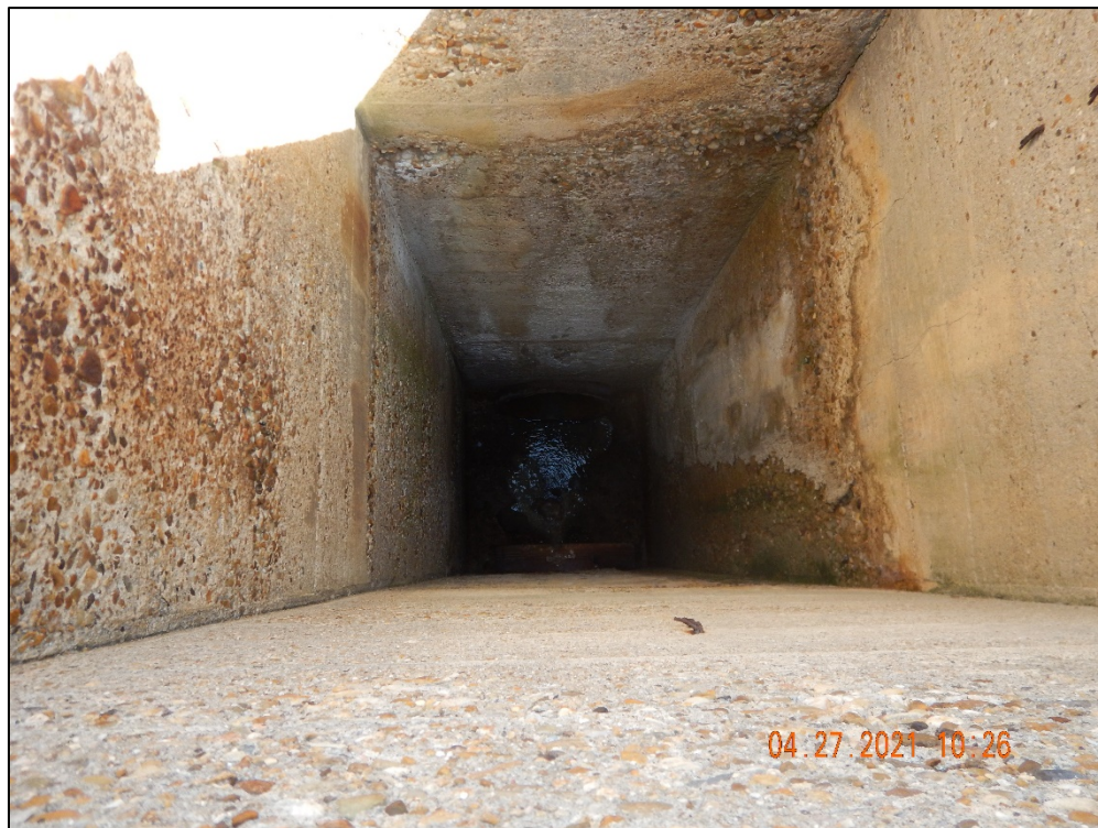
DSCN2321. View inside the sampling location for the Outfall 907 drainage area.
