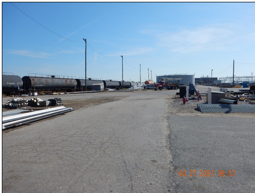
DSCN2307. View, facing east, of the equipment laydown yard in the Outfall 912 drainage area.
