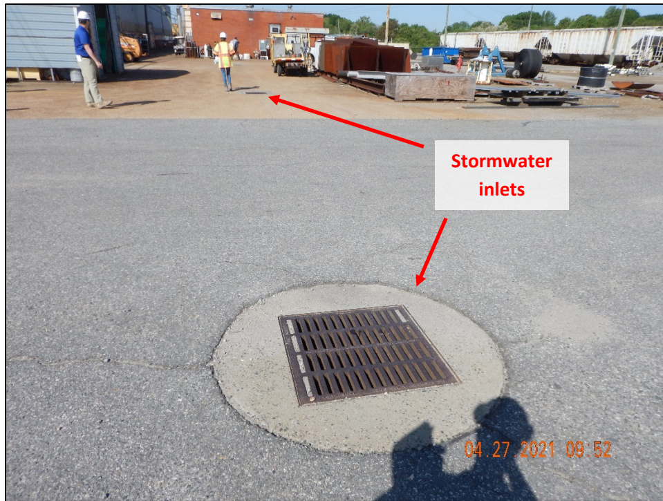
DSCN2305. View, facing west, of a stormwater inlet near the North Maintenance Shop, in the Outfall 912 drainage area.
