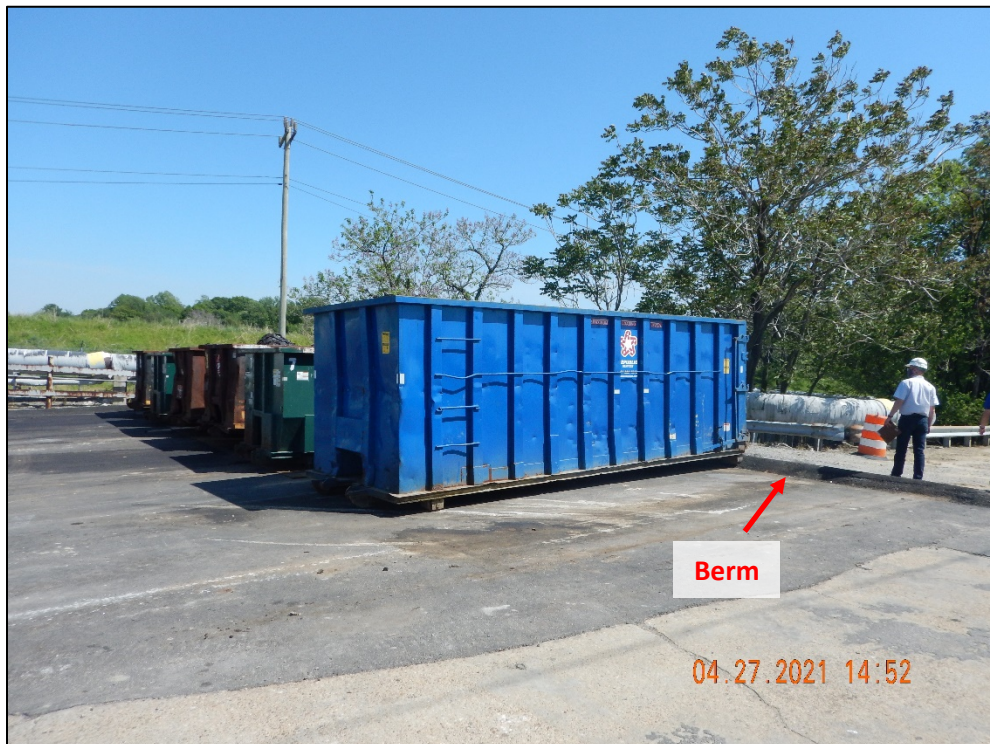
DSCN2386. View, facing southeast, of six uncovered dumpsters holding solid process waste. A berm had been installed behind the dumpsters to prevent runoff from reaching Outfall 910.
