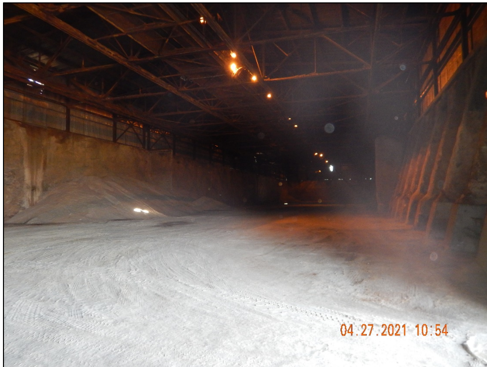
DSCN2330. View, facing west, of the inside of the ammonium sulfate fertilizer warehouse. Note the piles of fertilizer and heavy tracking throughout the warehouse.
