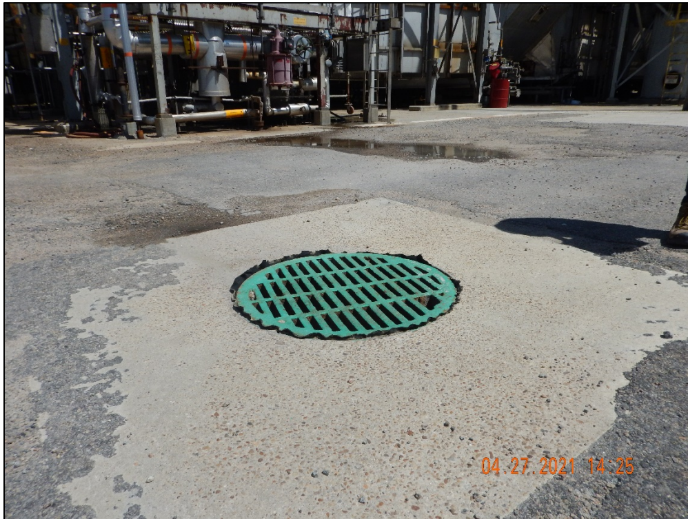
DSCN2380. View, facing southeast, of a stormwater inlet in the Outfall 003 clear water sewer system area.
