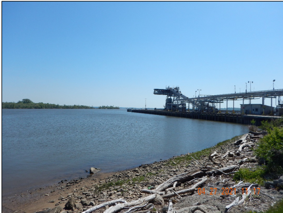
DSCN2341. View, facing southeast, of the Facility's large marine dock on the James River.
