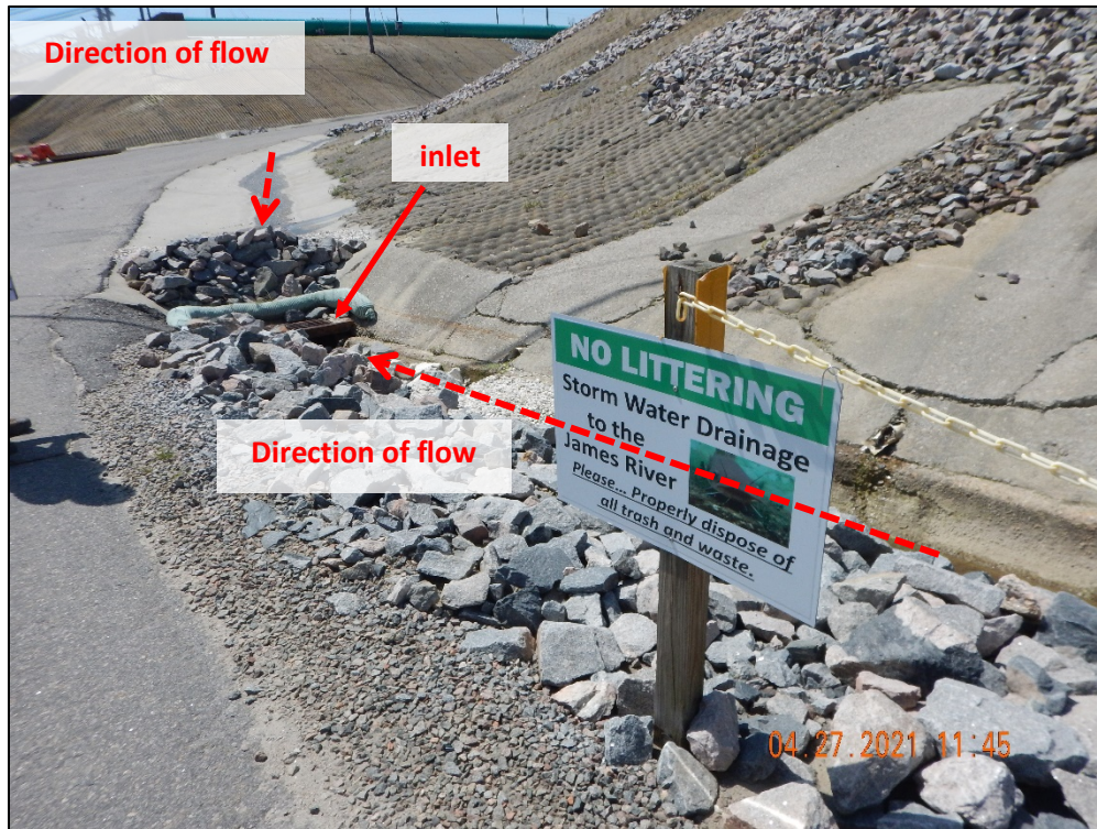
DSCN2352. View, facing south, of a storm inlet upgradient of Outfall 904. Note the rip rap and rolled inlet protection.
