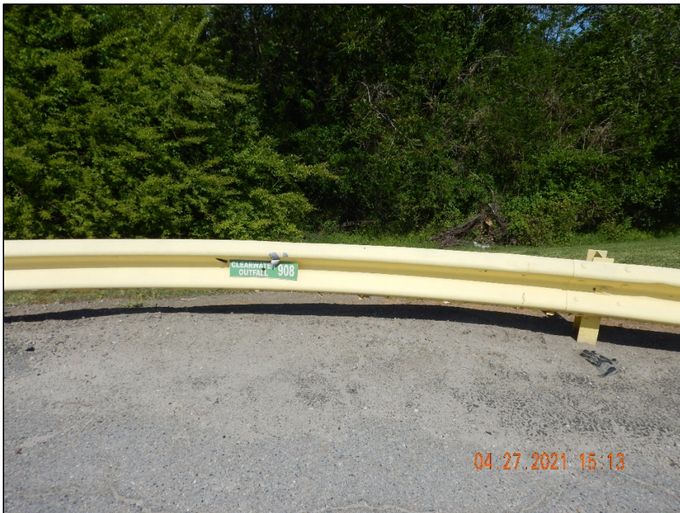
DSCN2396. View, facing north, of the wooded area containing stormwater Outfall 908. Outfall 908 discharges to Gravelly Run in the wooded area beyond the guard rail.
