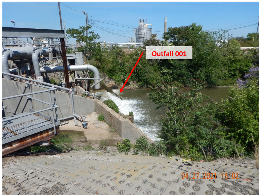
DSCN2391. View, facing east, of the large clear water sewer system Outfall 001. Outfall 001 drains stormwater, contact cooling water, and non-contact cooling water to Gravelly Run.
