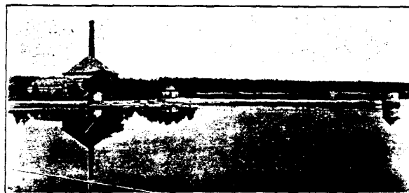
New Bedford pumping station and intakes on the shore of Little Quittacas Pond
