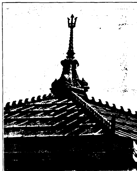
Detail of the impressive lead finial and lead-covered steel glazing bars used in the skylight; also lead cresting
