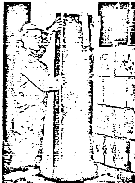
Courtesy of Lead Industries Association Mineralist Hermetat, Springfield, Illinois. A ray room is lined with 6-pd. sheet lead. The columns are also lined with sheet lead, while the walls are made of cinder block lead sandwiches.
