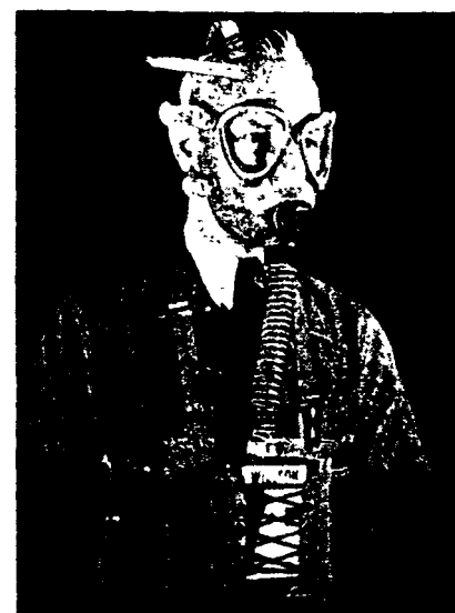
Fig. 5—Industrial gas mask (#1423) designed for protection against a specific type of vapor.
