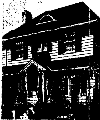
Now painting is needed to save costly repairs.
