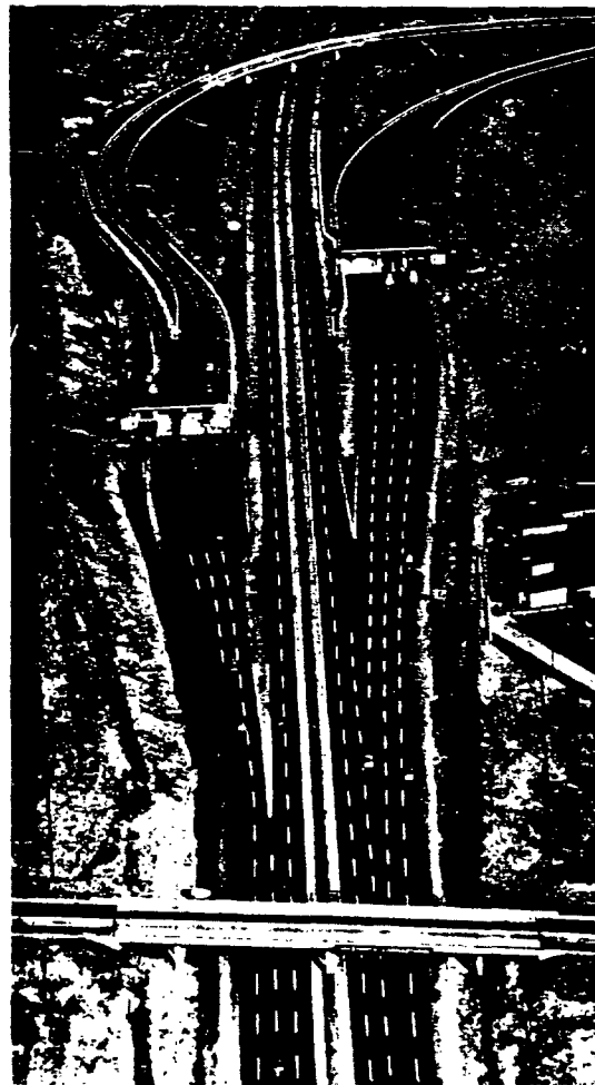
Asphalt's popularity zoomed when it proved so successful on heavily traveled turnpikes and expressways built soon after World War II.
