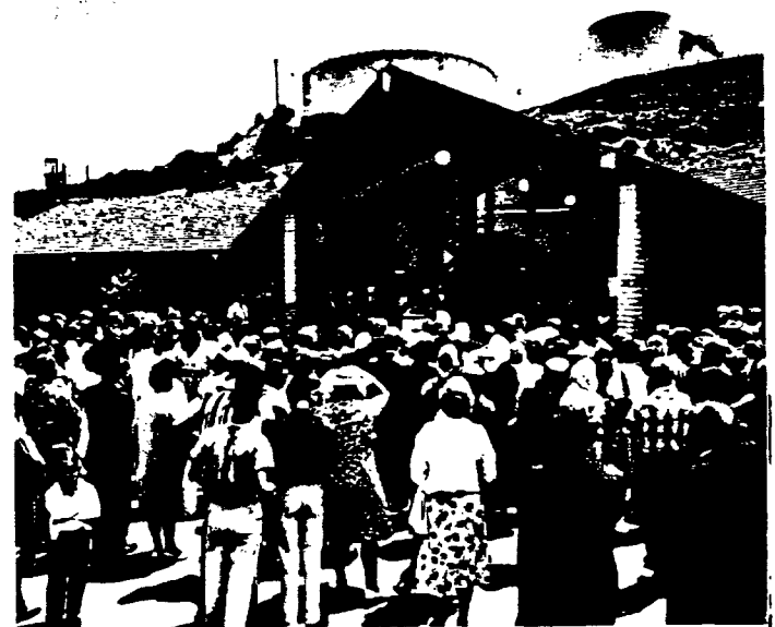
Active and retired Standard Oil Company of California employees gathered in front of the museum when it was presented to them by T. S. Petersen, then company president, last June. The 36-by-140-foot redwood and glass building is on the grounds of the Richmond refinery's Rod and Gun Club on the shore of San Pablo Bay.
