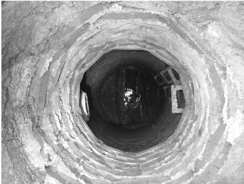
Photo 1: MH5363 (photo taken 10/2/2024 at approx. 09:39) Manhole located near the cross-section of Maginnis Ave and Sullivan Ave, discharging into the Merrimack River. Sample points are indicated by a red X.
