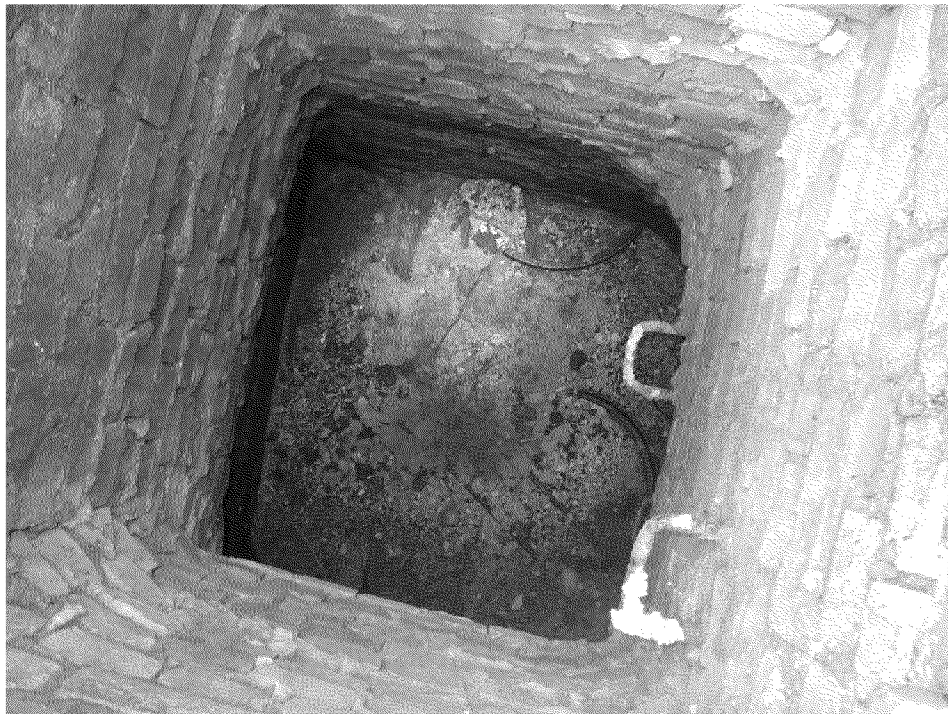
Photo 4: MH5275 (photo taken 10/2/2024 at approx. 10:53) Manhole located near Diamond St, closed off to receiving water.
