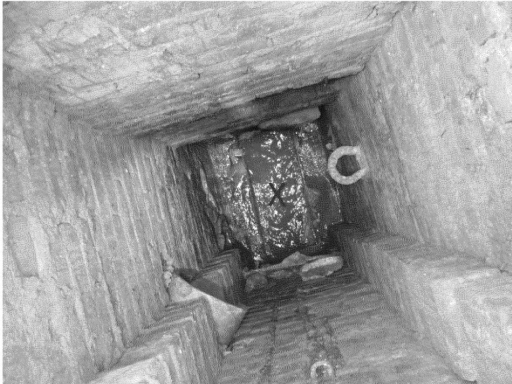
Photo 7: MH5503 (photo taken 10/2/2024 at approx. 12:55) Manhole located on Logan St, discharging into the Spicket River. Sample points are indicated by a red X.
