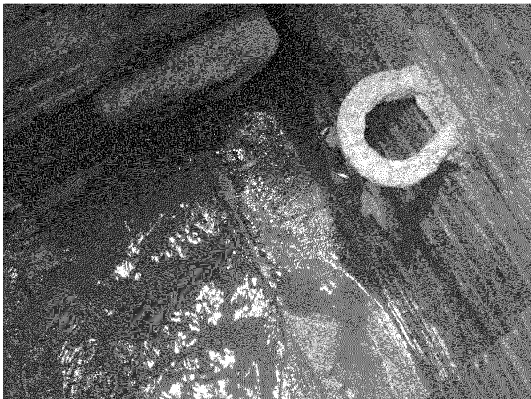
Photo 8: MH5503 (photo taken 10/2/2024 at approx. 12:56) Manhole located on Logan St, discharging into the Spicket River. Sample points are indicated by a red X.
