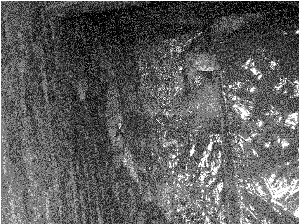
Photo 9: MH5503 (photo taken 10/2/2024 at approx. 12:56) Manhole located on Logan St, discharging into the Spicket River. Sample points are indicated by a red X.
