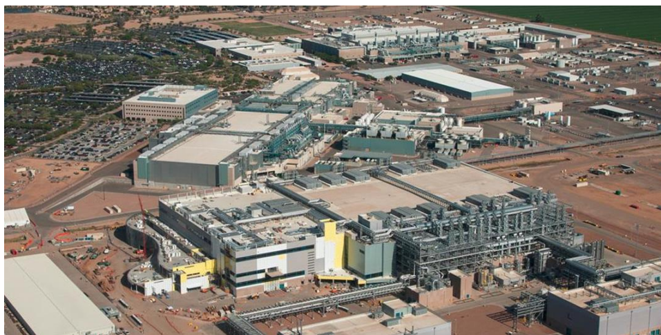
Figure 18: A semiconductor manufacturing facility (Intel 2017).
