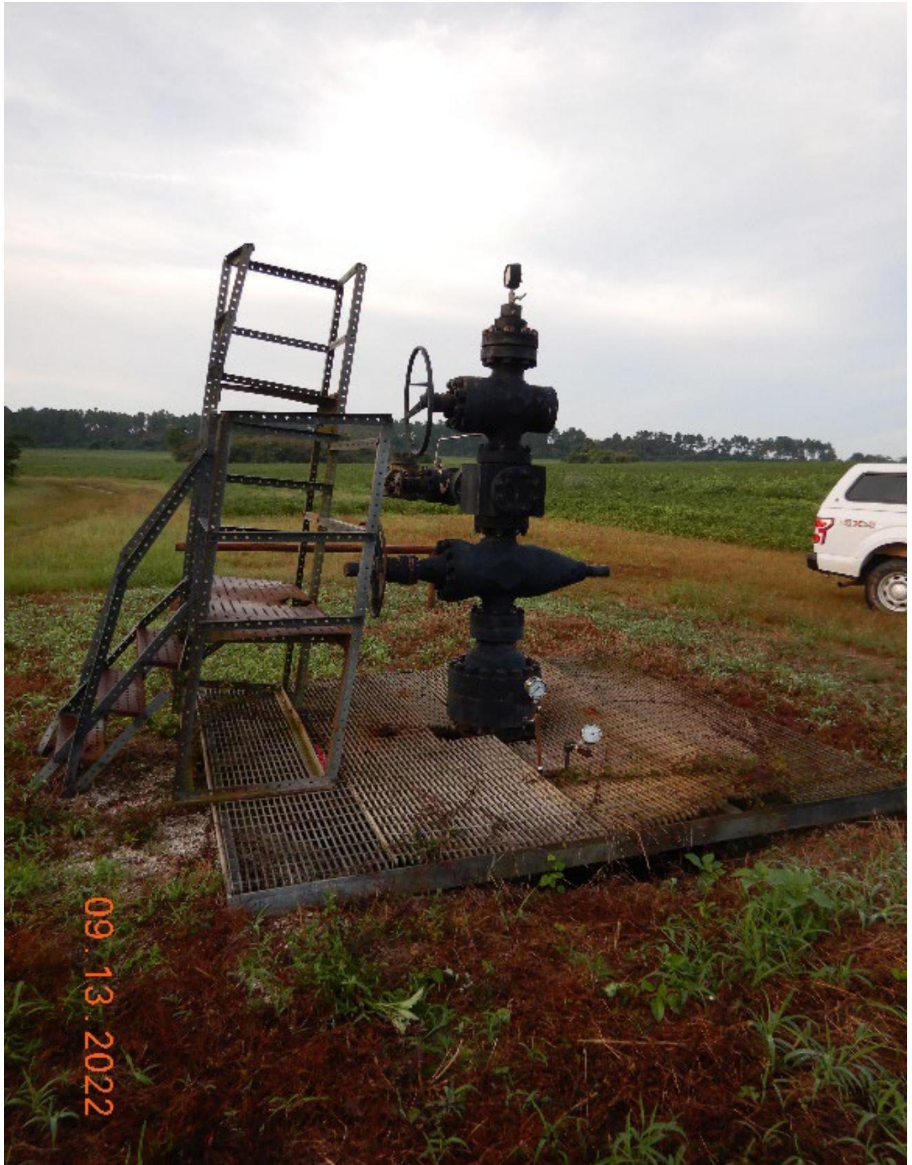
Photograph 2: Looking south, site overview, including well head, pressure gauges, valves, and access stairs.
