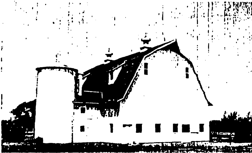
Figure 53.—This dairy barn is repainted every 5 years as part of a regular painting program. Such a practice is followed by many successful farmers.
