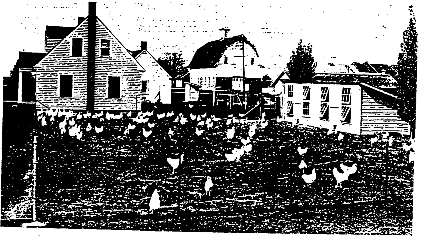
A sure sign of a progressive farmer—well painted buildings in attractive and well-kept surroundings.
